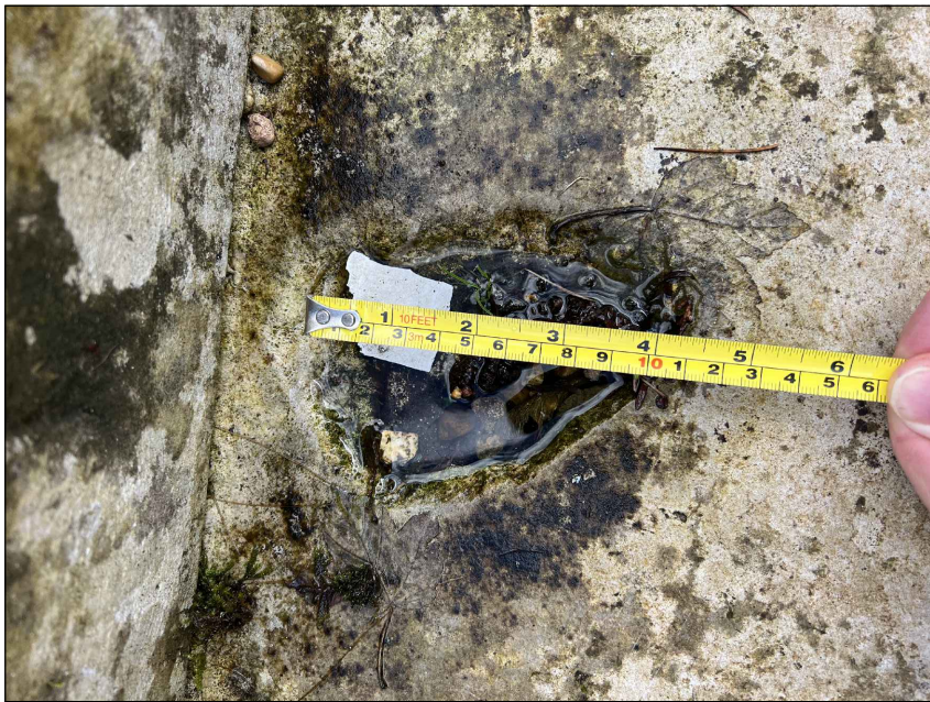
Photo 3 - Nominal 110mm depression in stone surface
