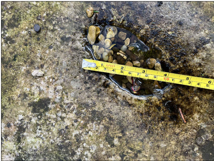
Photo 4 - Nominal 110mm depression in stone surface
