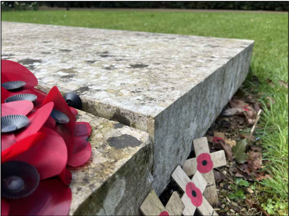
Photo 9 - Stones misaligned at joint
