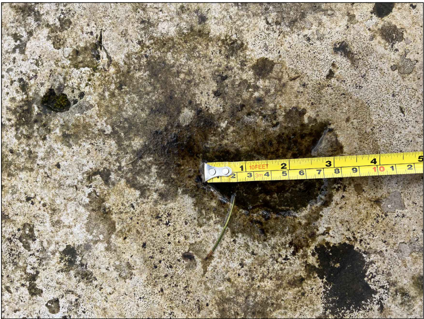
Photo 2 - Nominal 80mm depression in stone surface
