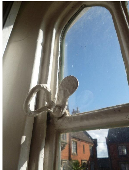
Iron thumb & pivot window stay catch.
