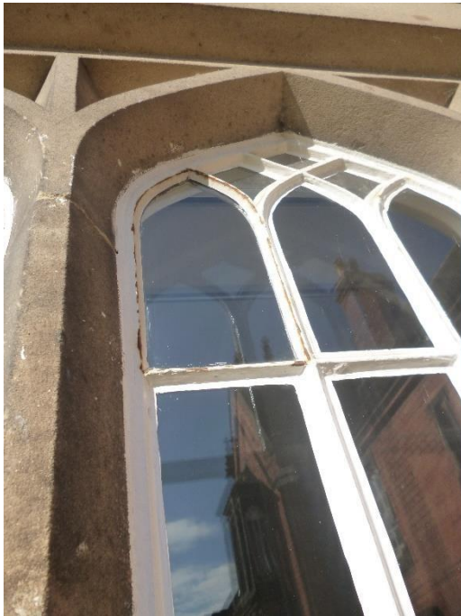
Corroding window frame edges.
