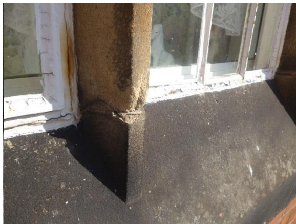
Mullion seating and base of mullion weathering and split.
