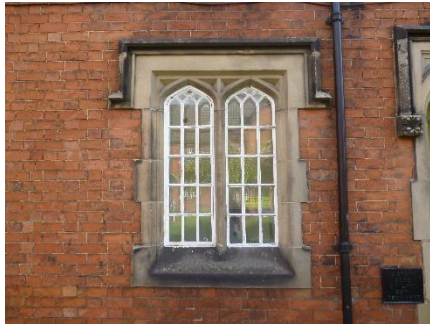
Broken window pane to opening casement
