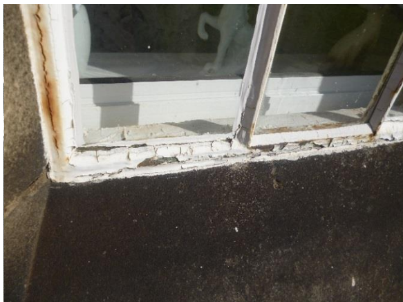
Paint coating failing and corrosion coming through.
