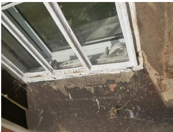
Window stay with scroll detail visible behind opening casement.
