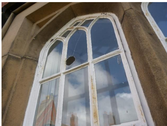
Broken window pane to opening casement
