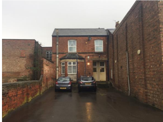
Fig. 05 View of rear block from car park.
