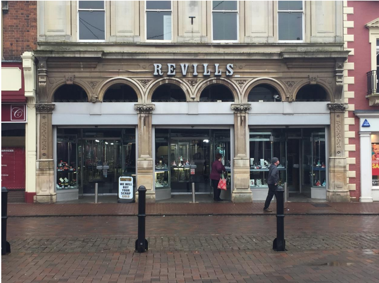
Fig. 15 The north-east elevation at ground floor level as it exists in 2017.
