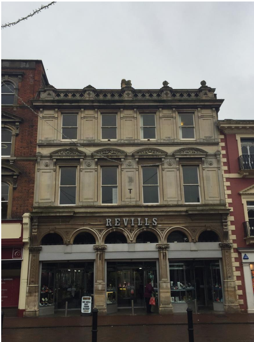
Fig. 03 Frontage elevation (north-east) to the Market Place
