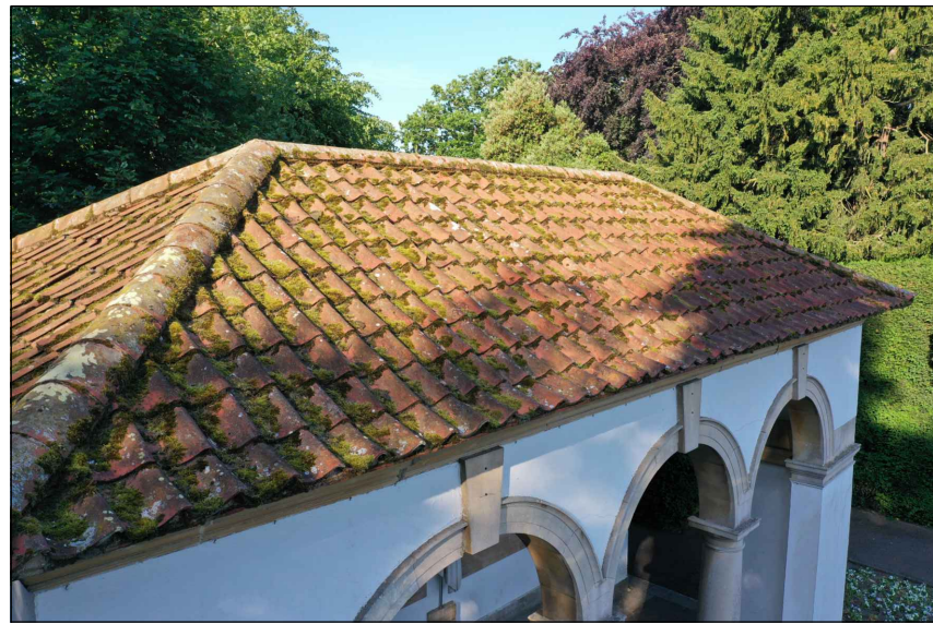
Photo 5 - roof level view of War Memorial from north-east
