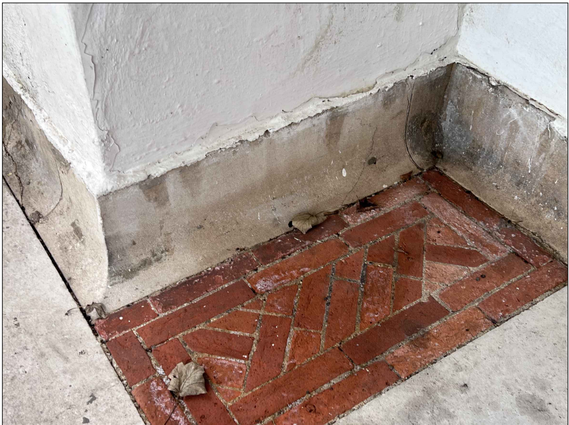
View of Brick Panel 2 from north. Scheduled for DOFF clean and repoint only.
