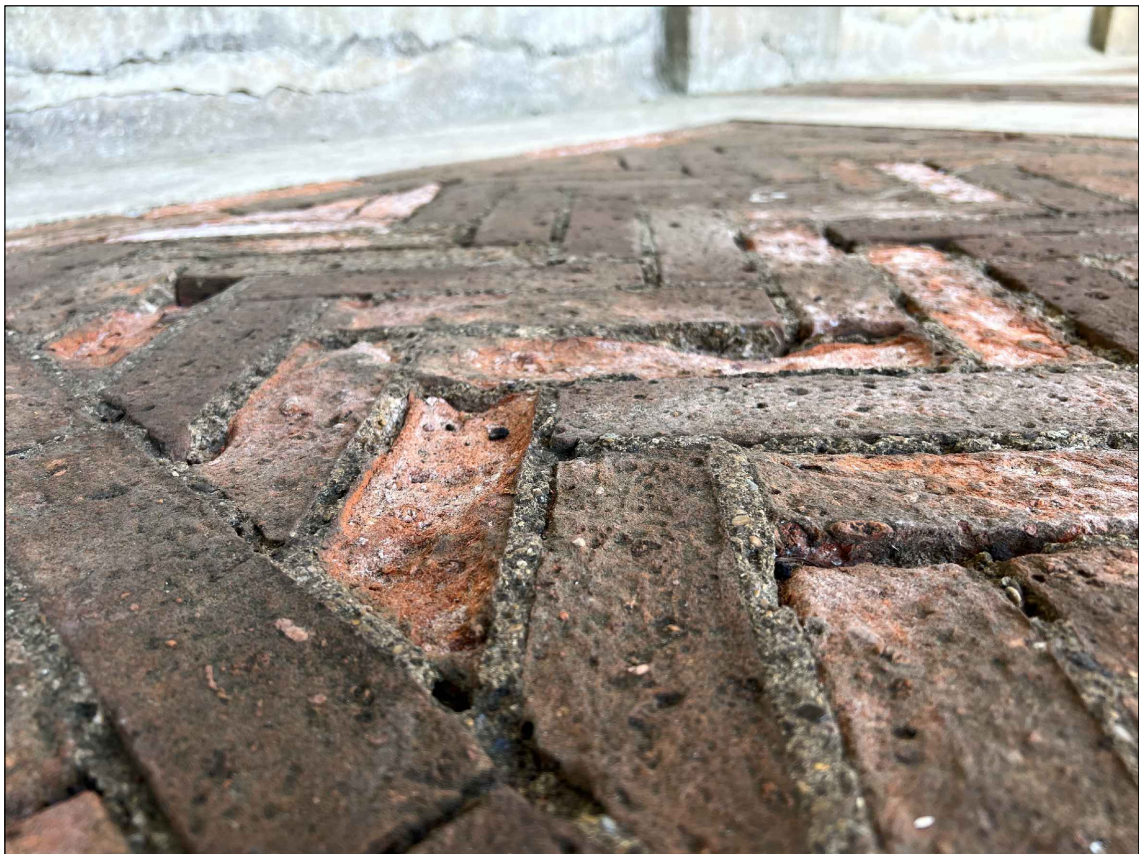
Detailed view of damaged brick surface in Brick Panel 4. Scheduled for replacement of bricks, DOFF clean and repoint.
