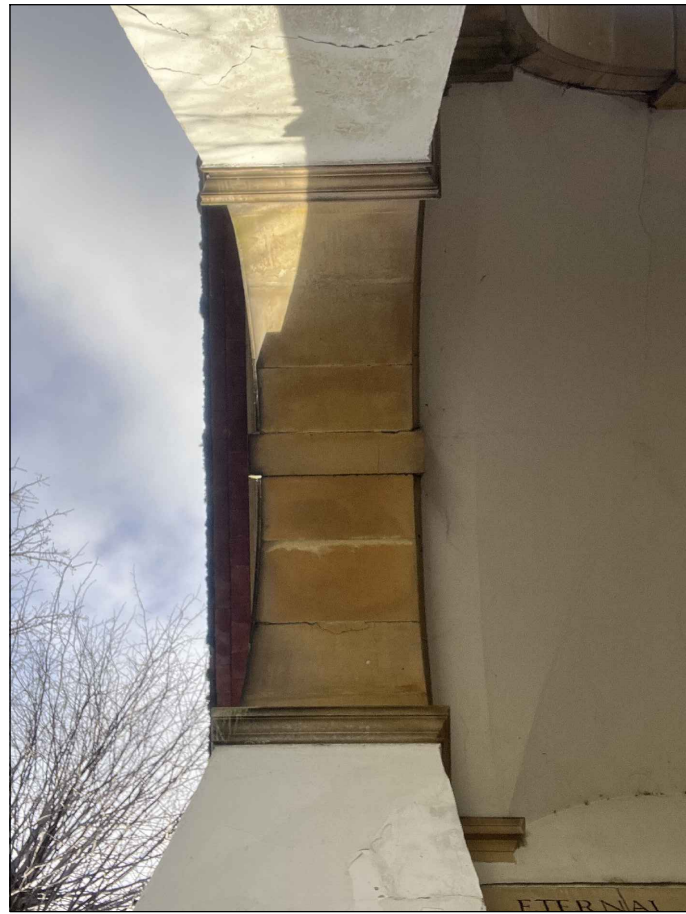
Ceiling view - Arch 1
