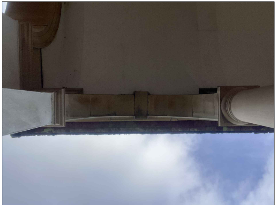
Ceiling view - Arch 4
