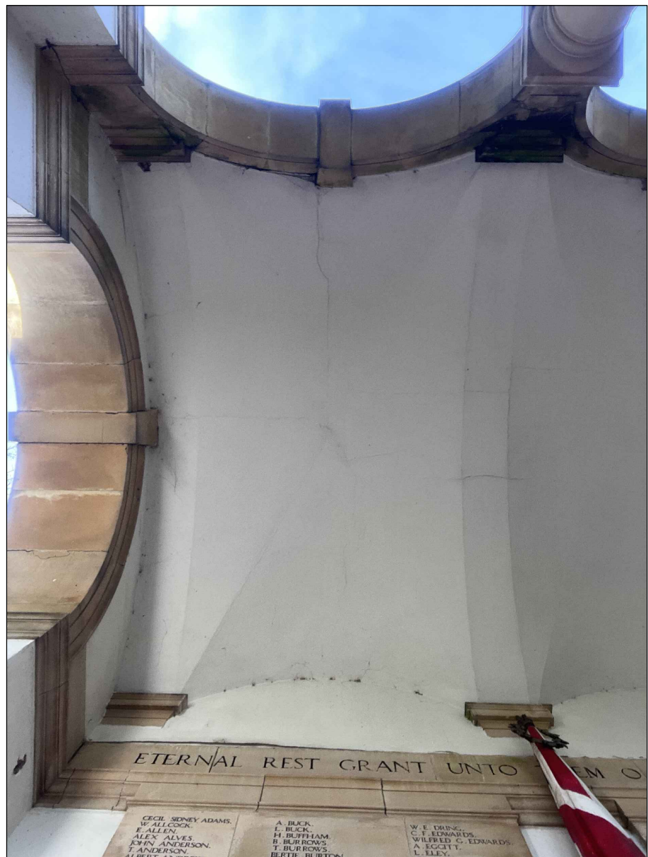
Ceiling view - East Vault
