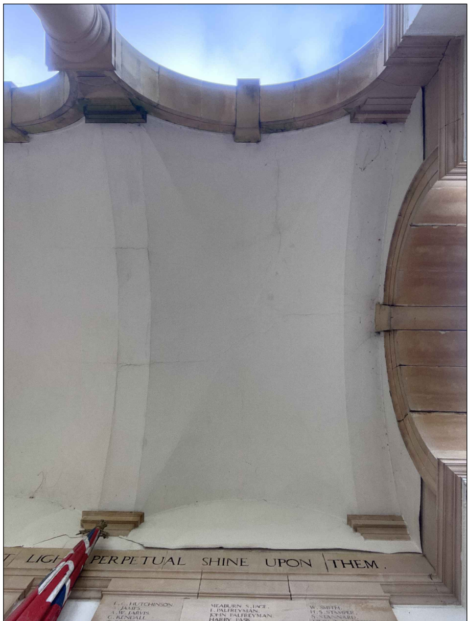
Ceiling view - West Vault
