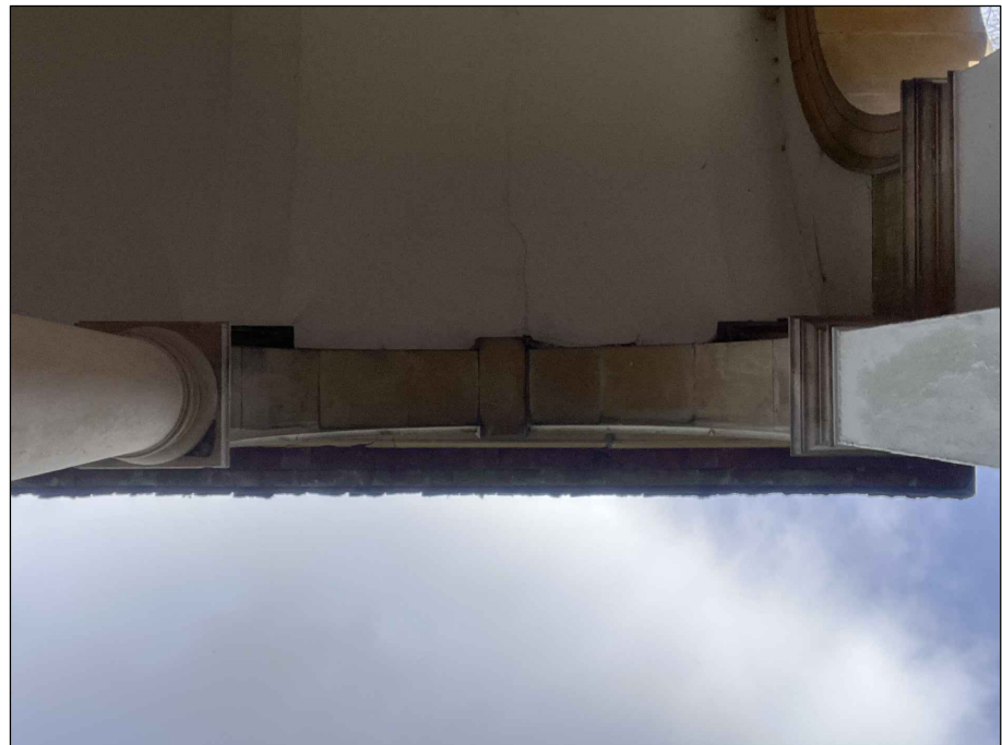
Ceiling view - Arch 2
