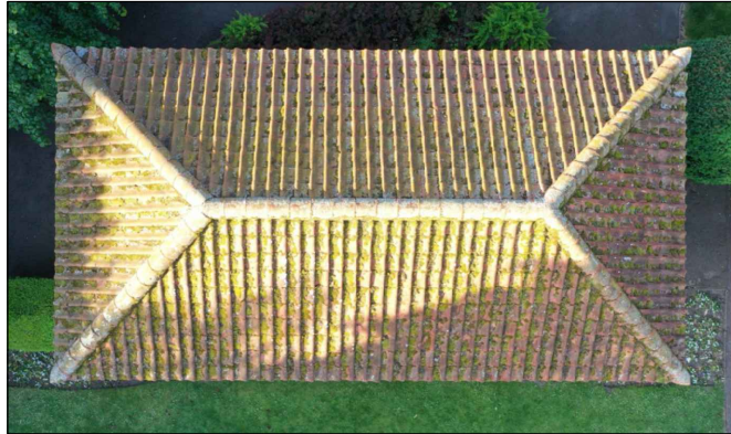
Aerial view of roof
