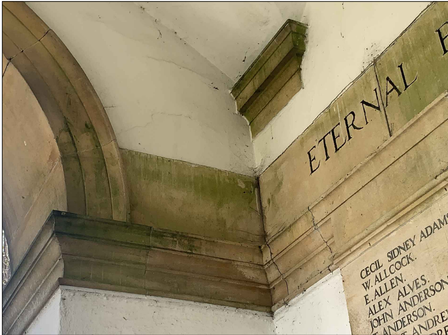
Image of stone cornice, frieze and corbel
