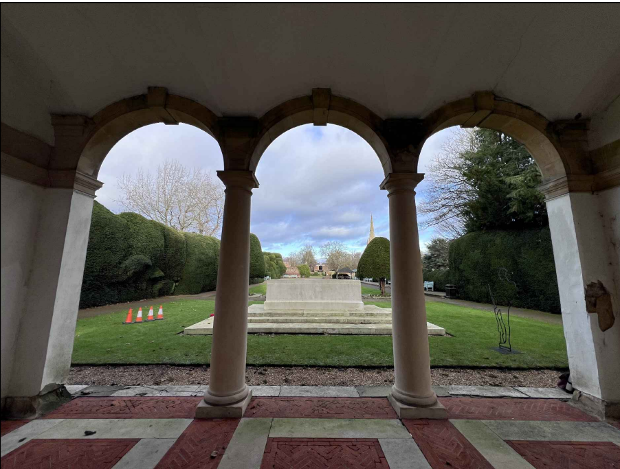
General view of arches 4, 3 and 2.
