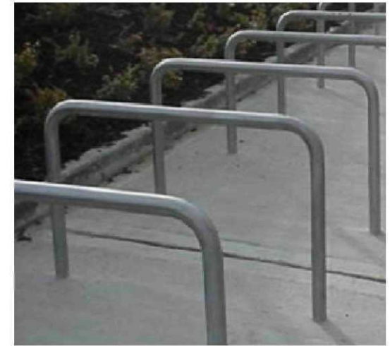
Example of proposed stainless steel cycle hoops
