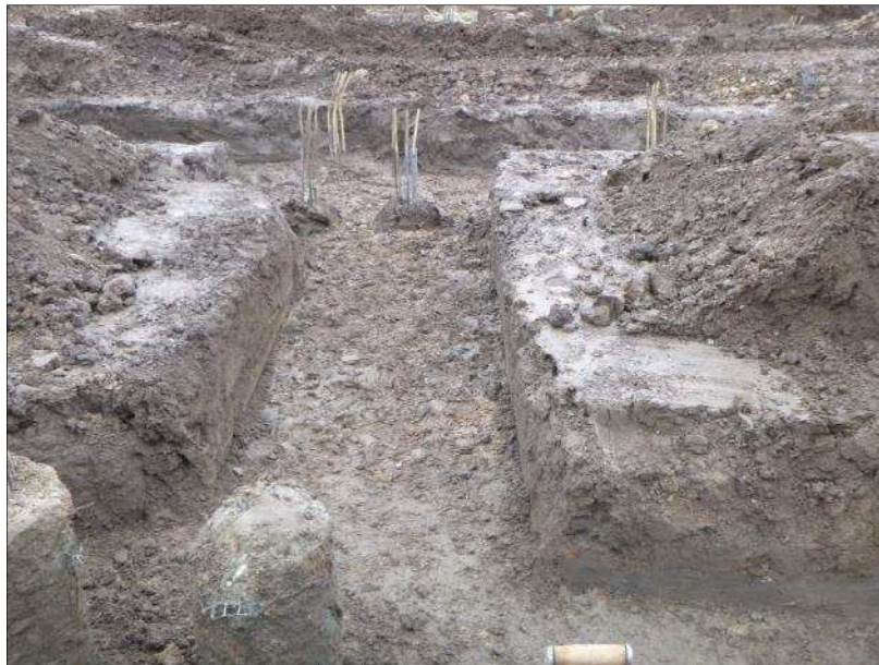
Plate 2: View of the southern end of site looking west, showing imported soil 104 and buried topsoil 105
