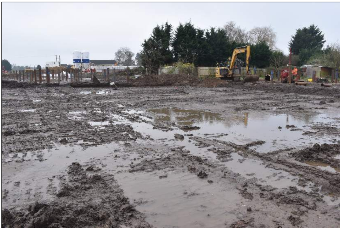
Plate 2: Pre-excavation view across Area A, looking southwest
