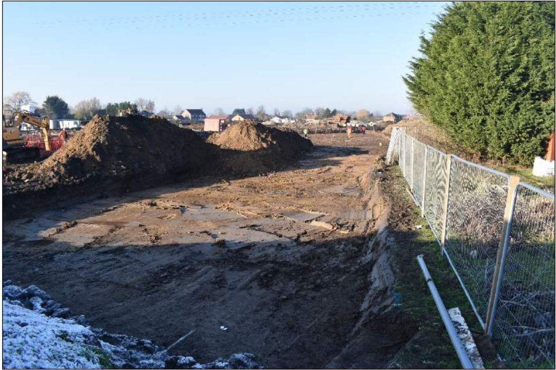
Plate 19: View of Area B from the south, looking north
