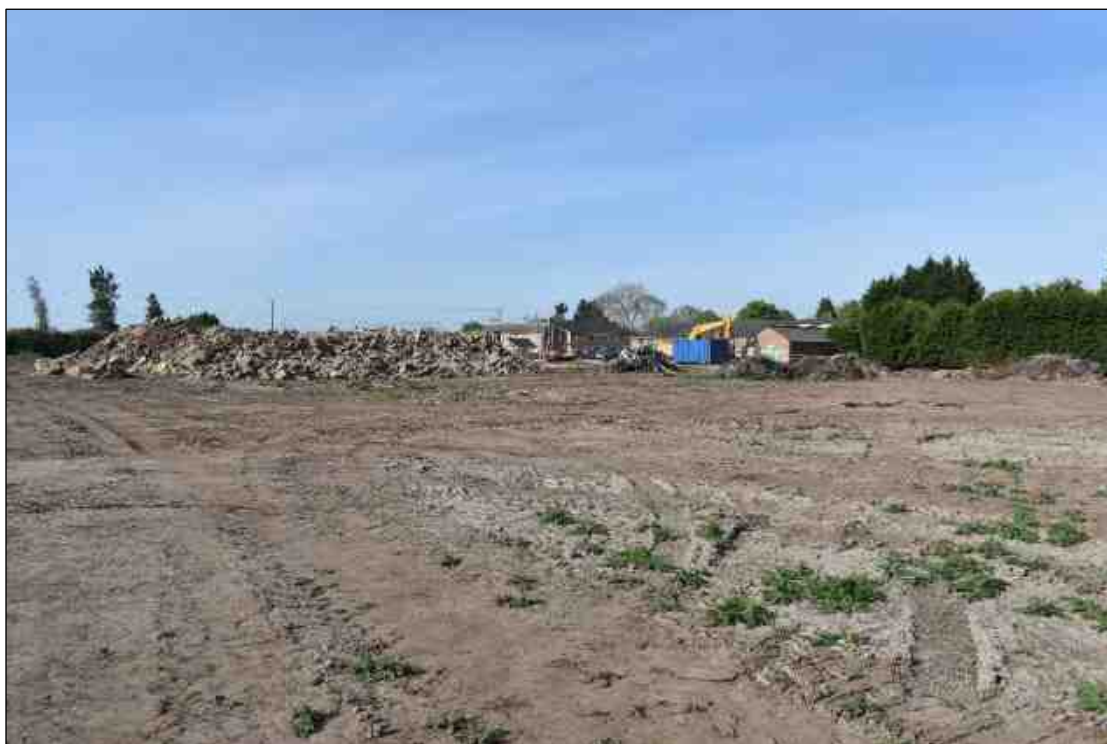
Plate 4: North end of the site, looking southwest
