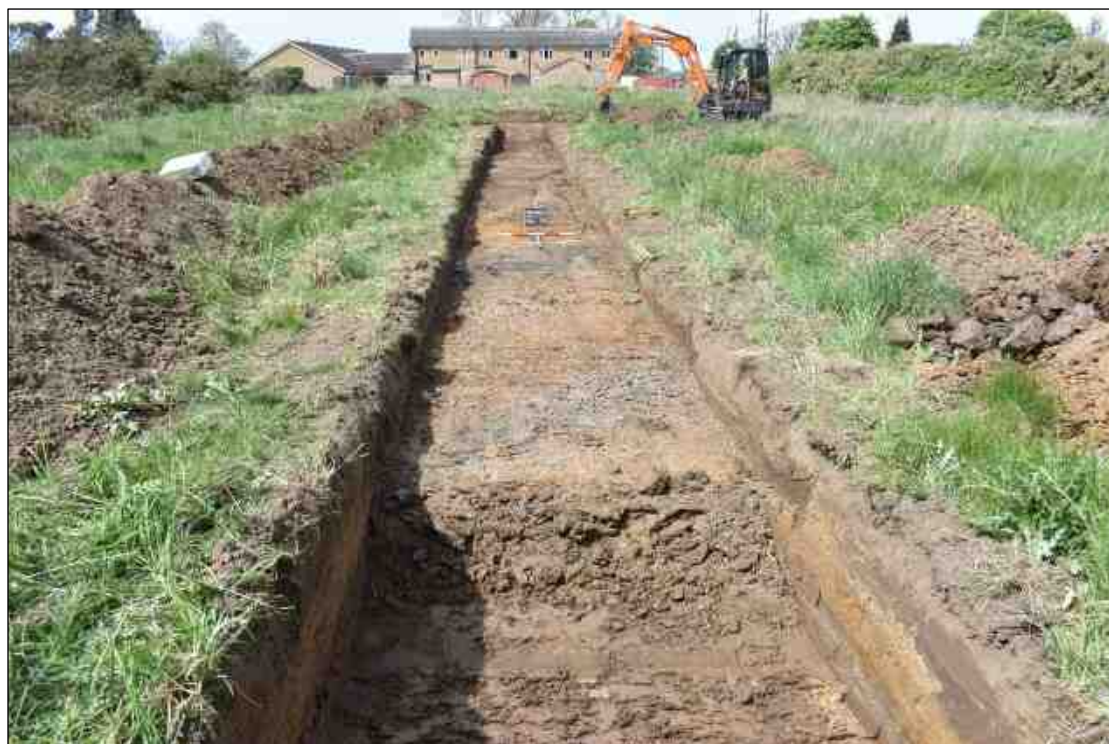
Plate 21: Trench 16, looking west
