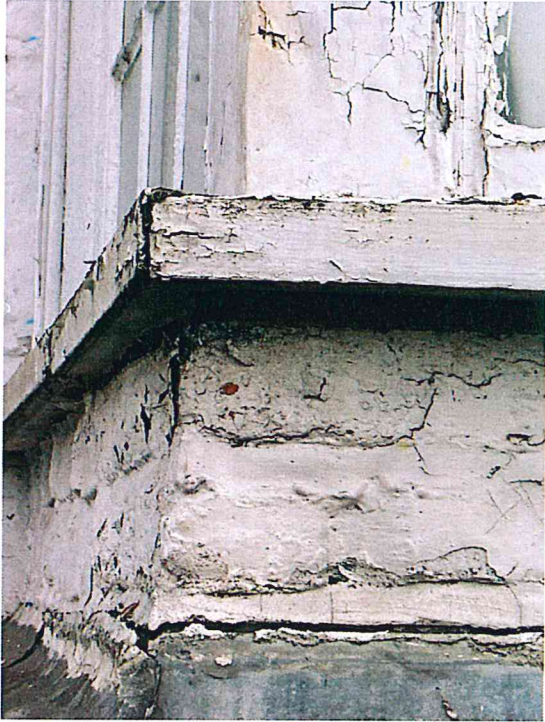
Image showing clear movement of FF Bay window
