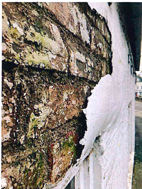
Paint blown from bricks
