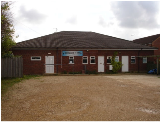
Existing premises in Horseshoe Road, Spalding
