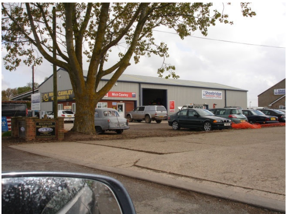
Mick Cawley/Shoebridge Engineering (Kellet Gate)
