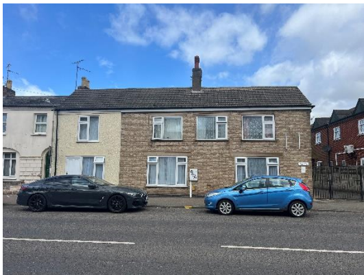
Fig. 01 – View from Westlode Street
