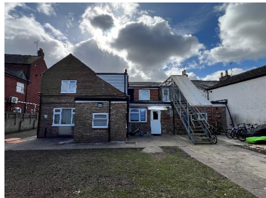
Fig. 02 – View from the rear
