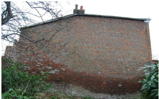
Fig 10. Gable end wall of No 12 Church Gate
