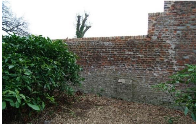
Fig 11 Shows the start of the wall that has been reduced in height
