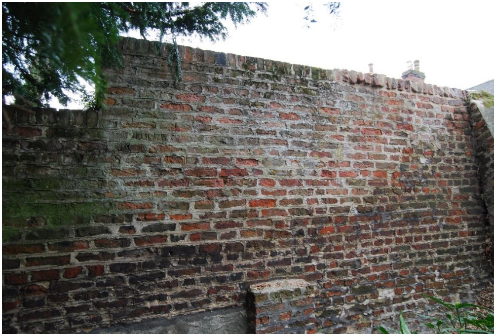
Fig 17 Left of the rendered buttress where the new header course meets the existing.
