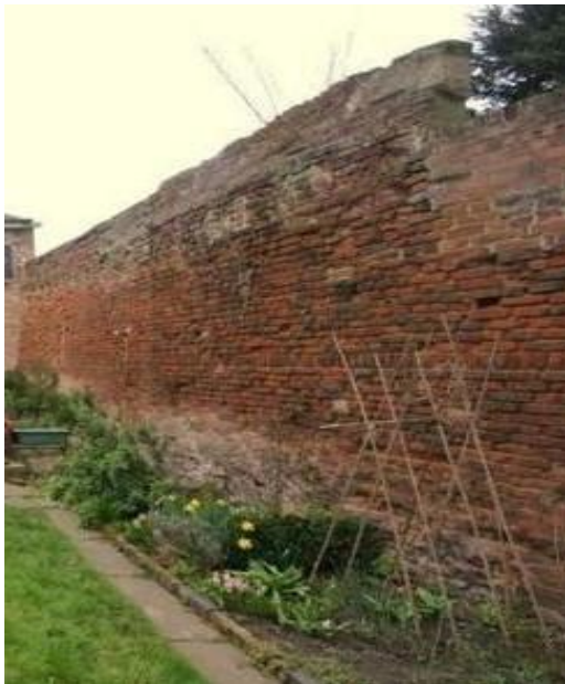
Fig 14 Original height of wall prior to reduction
