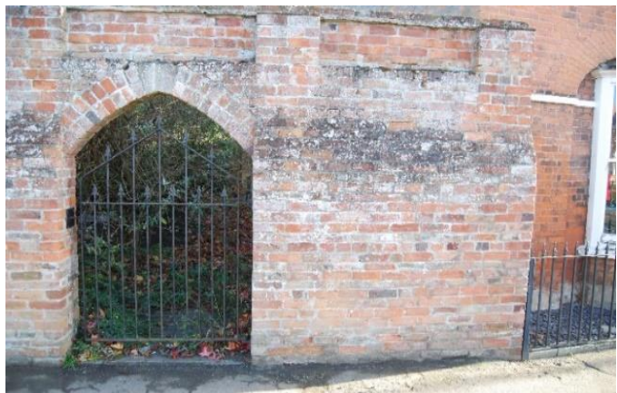
Fig 8. View of the gate to Ayscoughfee Gardens adjacent to No12.viewed from Church Gate
