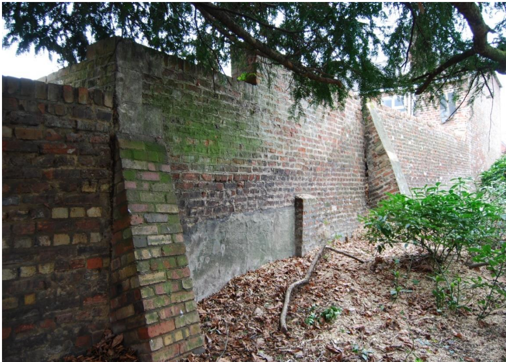
Fig 18 View showing where the unaltered section of wall meets the rear garden wall
