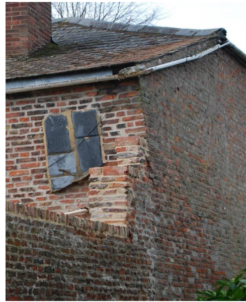
Fig 15 Wall at junction of house showing thickness
