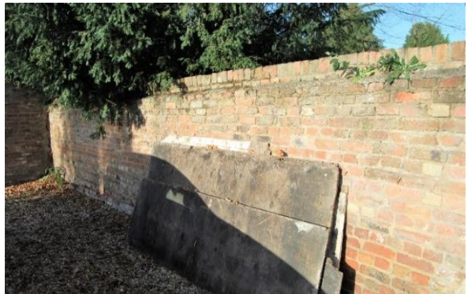
Fig 12 Area to the rear of No 12 Church Gate mentioned in 5.1.3 above
