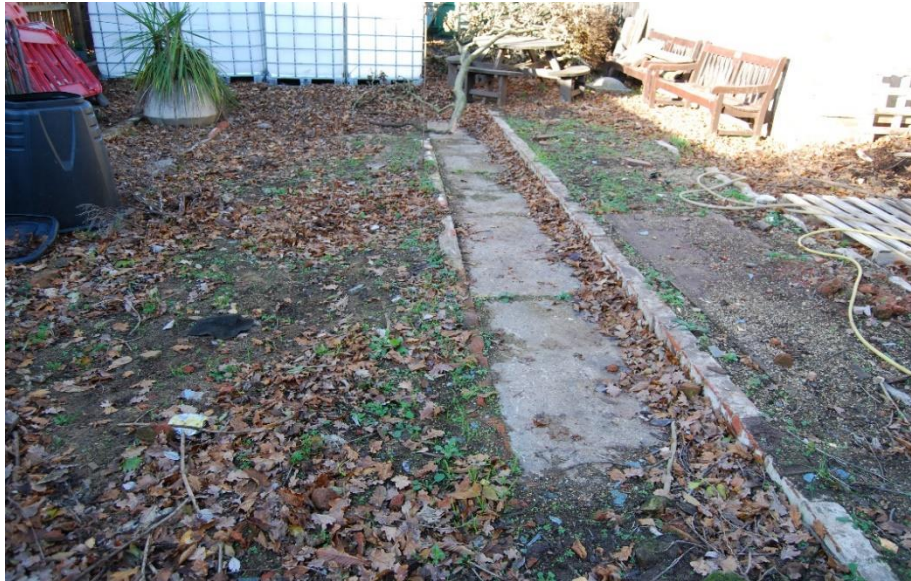
Fig 12. Image showing the bases of the Greenhouses December 2021
