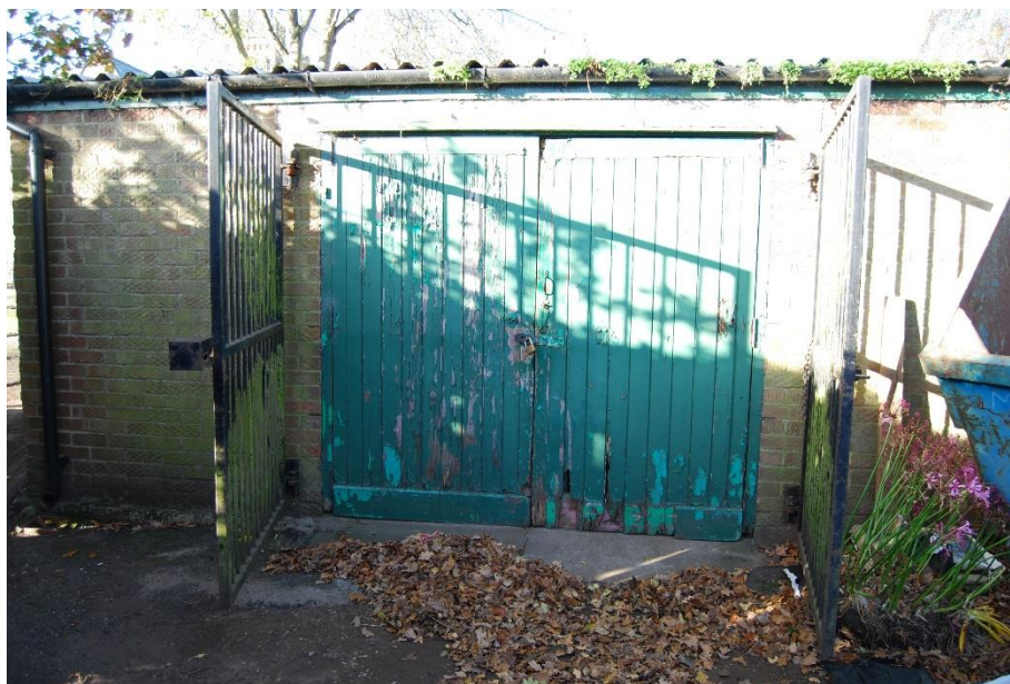
Fig 15 The doors to the Gardener's store which are to be removed and replaced with a roller shutter door
