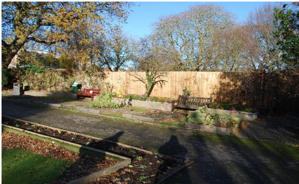
Fig 9. View of the fence viewed from the bowling green, showing the older section to the left and the new length erected on the same line, to the right
