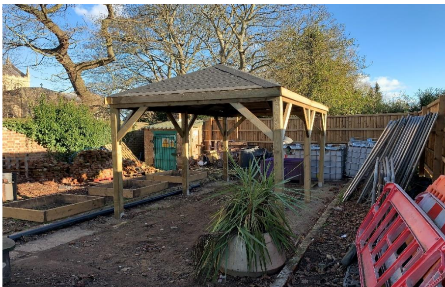
Fig 13 The free standing shelter April 2022
