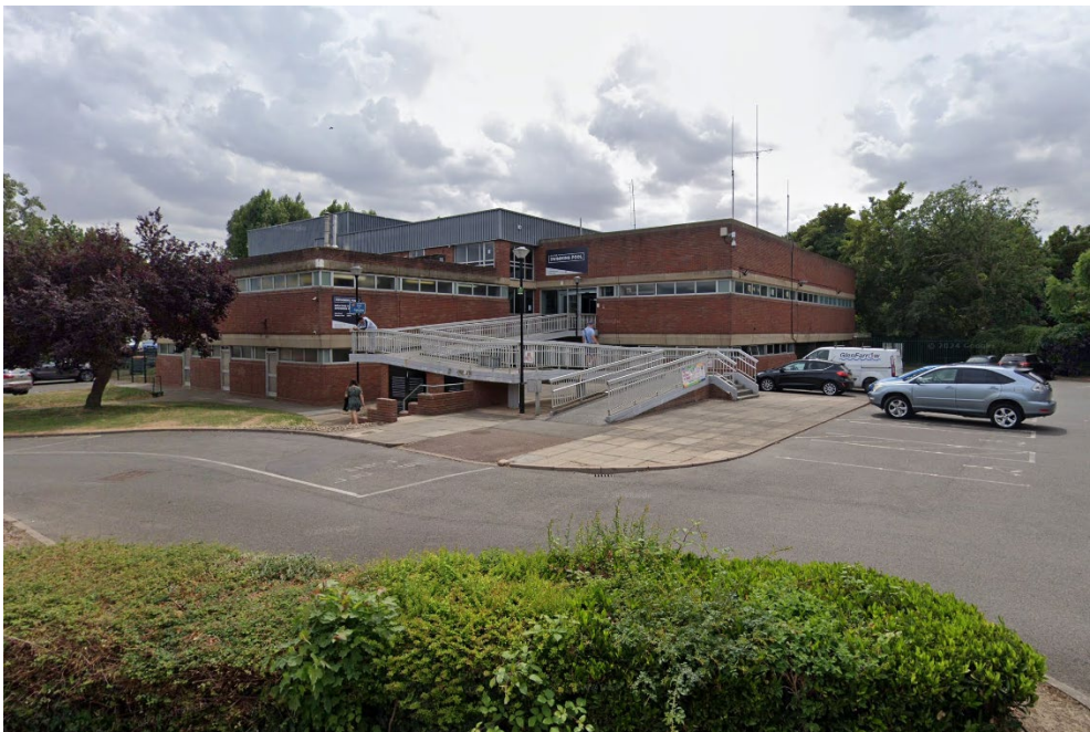
View of the front of the existing swimming pool
