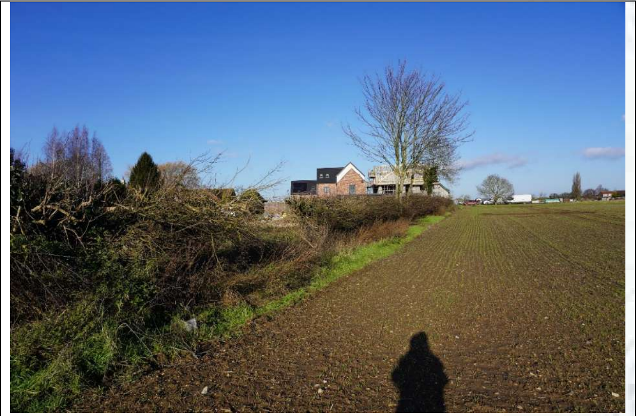
Plate 23: View north from the south-west corner of the Site towards Horseshoe Road and the house under construction
