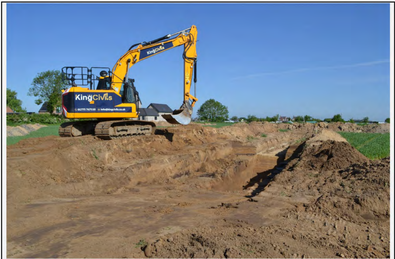
Plate 22 – Trench 12. View of additional machine excavation, looking northwest
