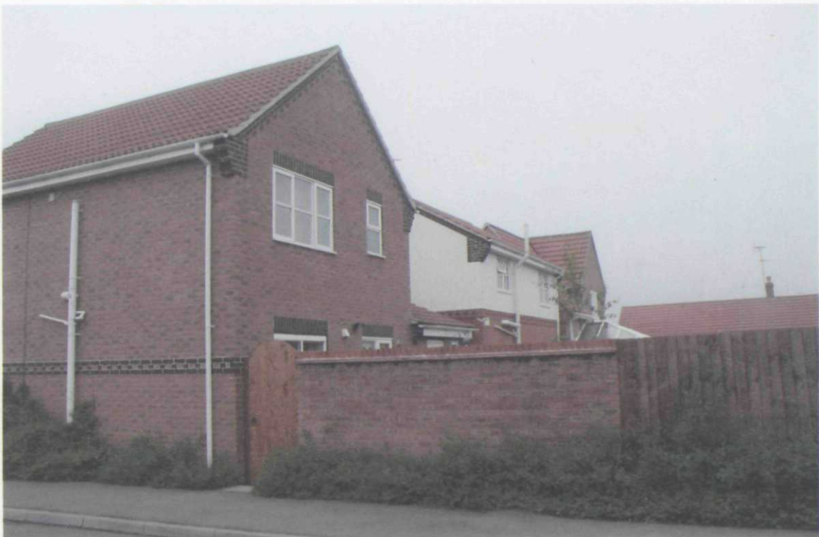
Rear of no 10 & no 9.
