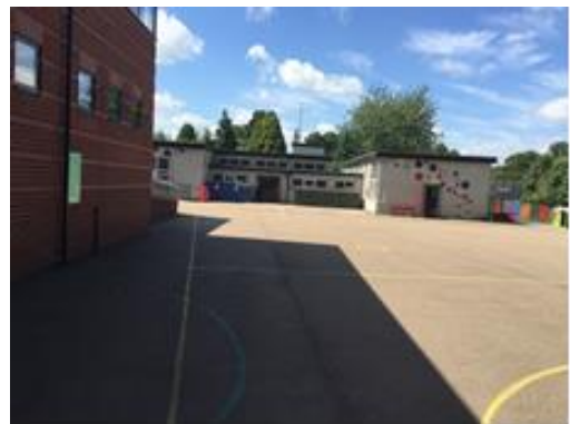
Fig. 02 – Annex block in the west corner of the site.
