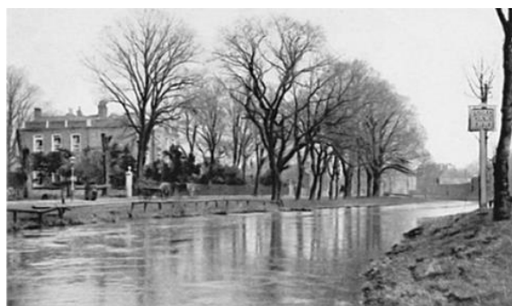
Fig. 15 – Photograph taken from Cowbit Road shows Welland Hall, London Road on the left and River Welland (date unknown). Sourced from http://www.southhollandlife.com/category/spalding
