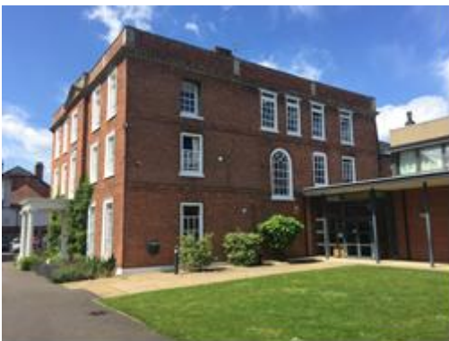
Fig. 01 – The original Welland Hall Building (main school premises).
