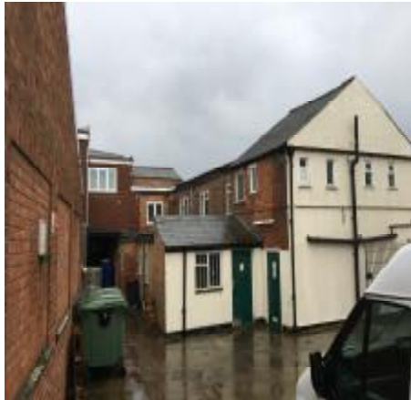
Fig. 07 – Side / rear elevation taken from rear courtyard
