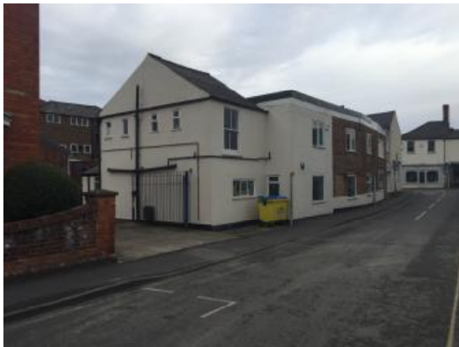
Fig. 02 – View from Priory Road towards The Crescent
