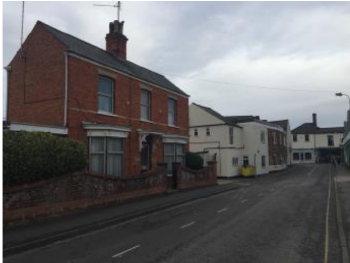
Fig. 03 – View from Priory Road towards The Crescent
