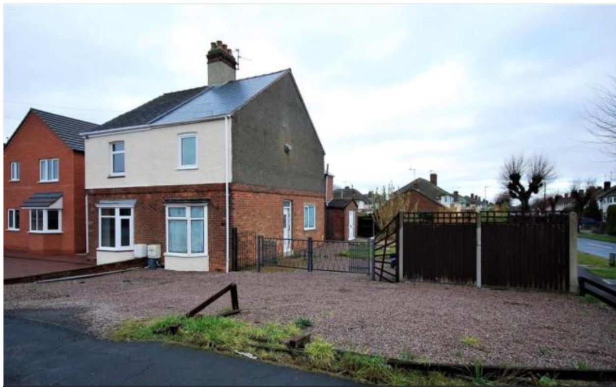
PIC 3 Parking at front of dwellings
