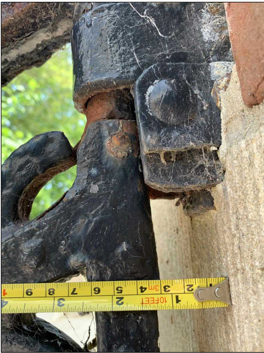
Fixed hinge point on south pillar
