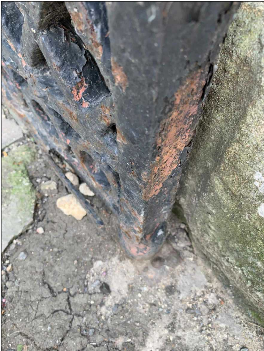
Ground-mount pivot point at south pillar
