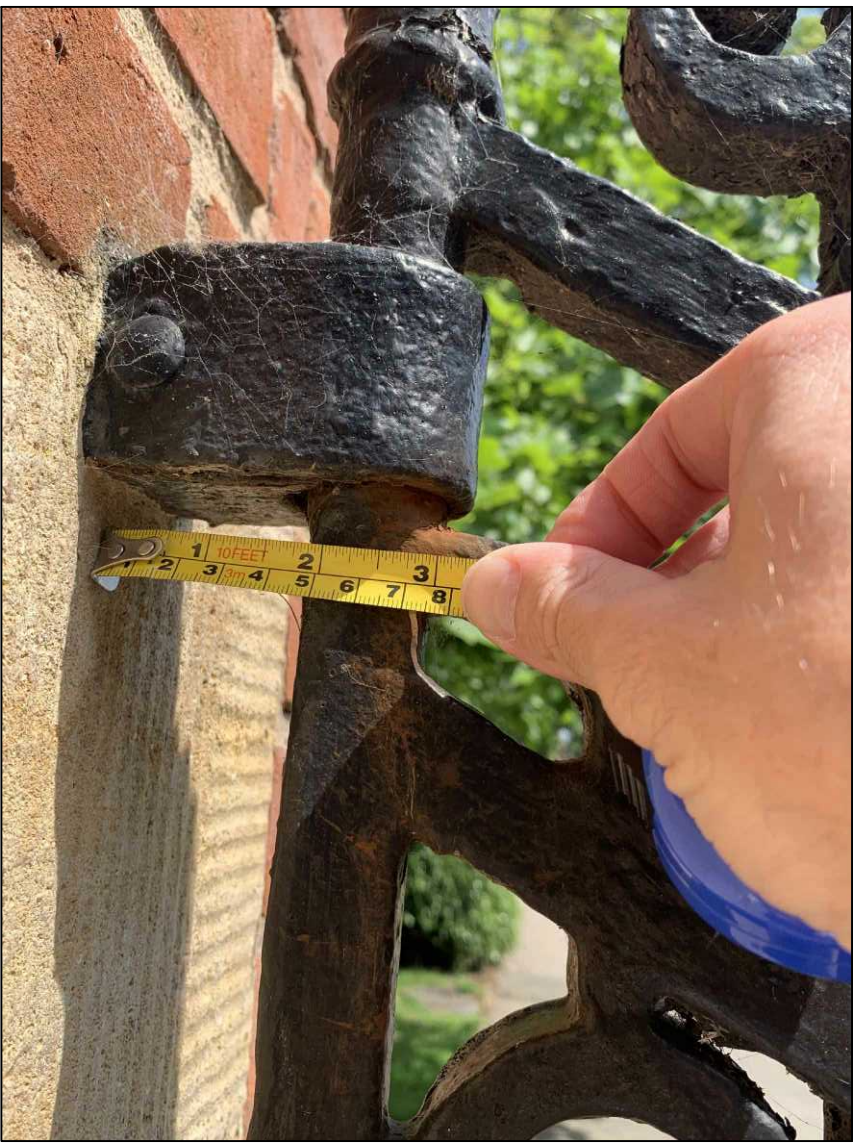
Fixes hinge point on north pillar
