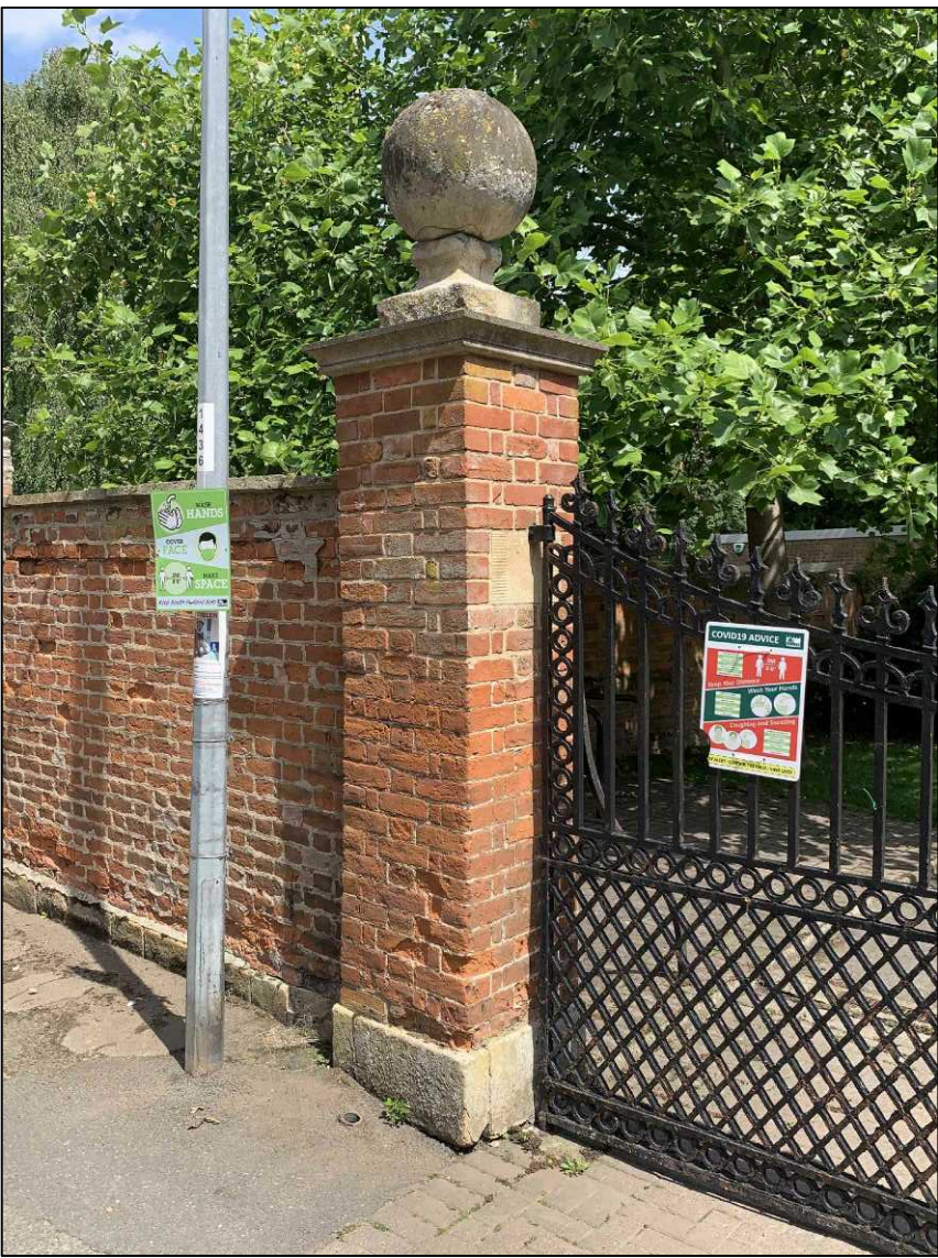
North pillar - top section rebuilt
