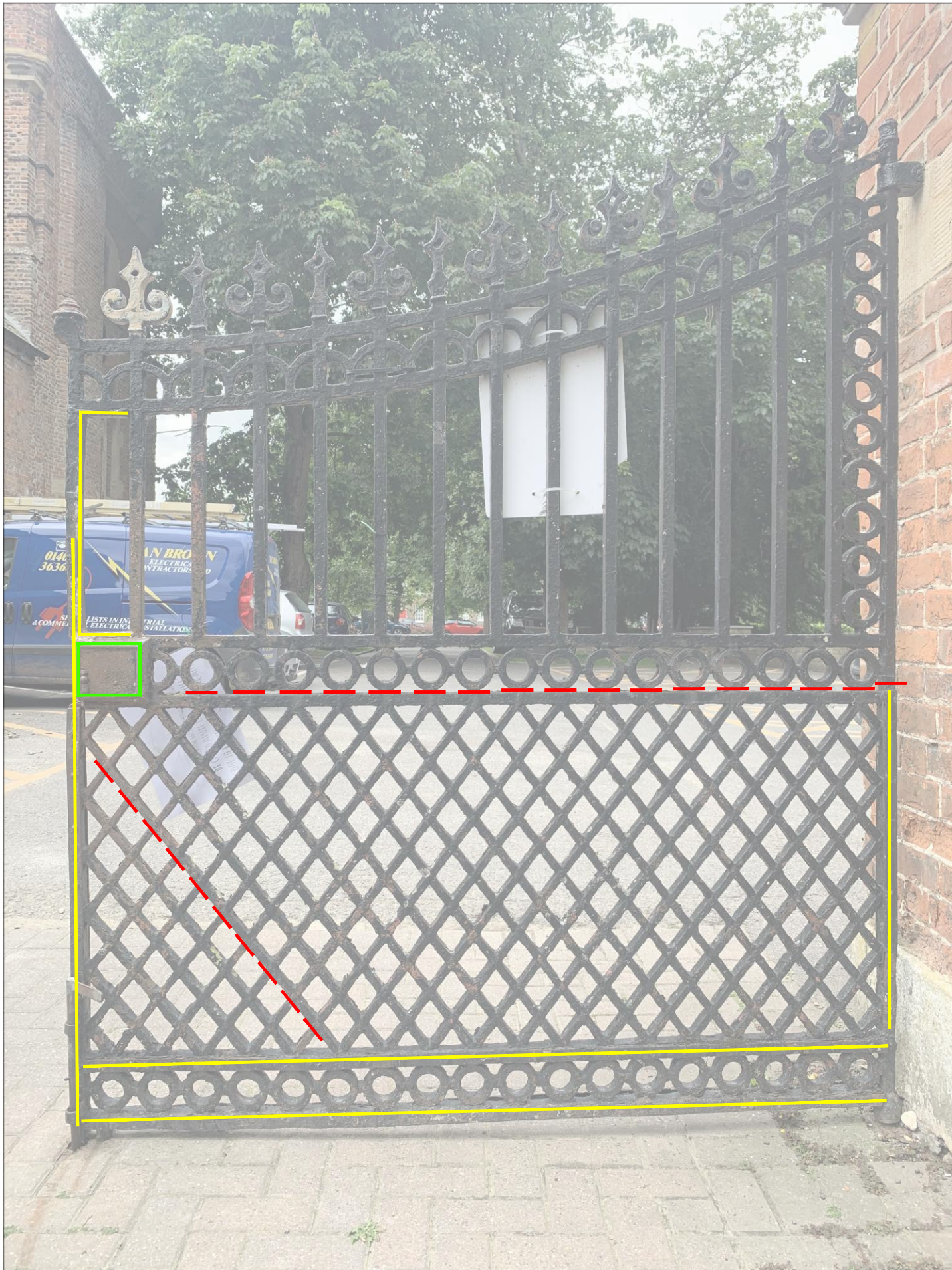
North gate (from east)
