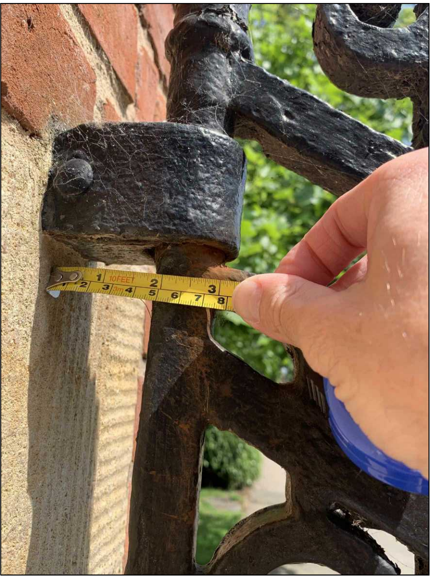
Fixes hinge point on north pillar
