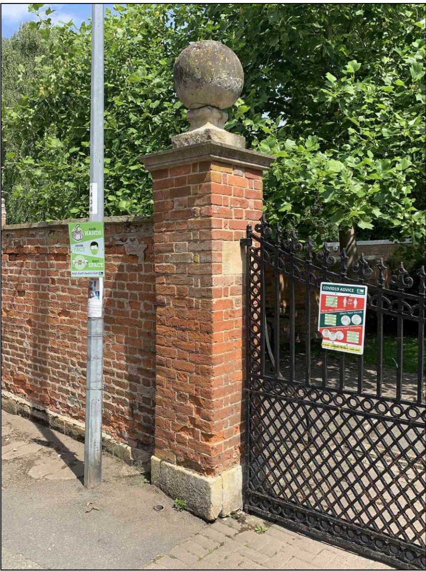
North pillar - top section rebuilt
