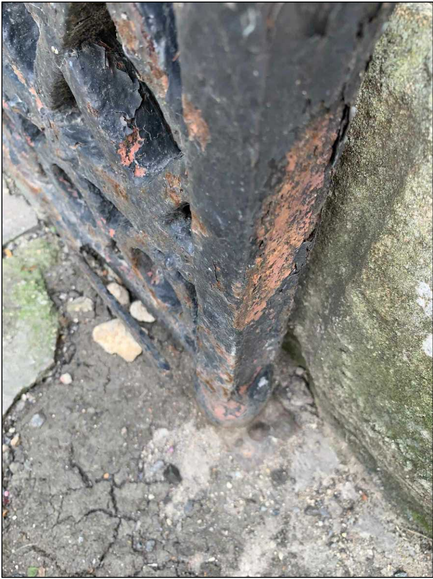
Ground-mount pivot point at south pillar
