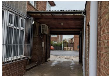
4 - Covered underpass / Bourne Road
