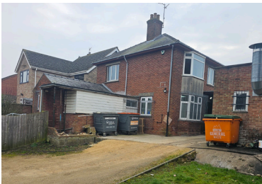
3 - rear extension / slope
