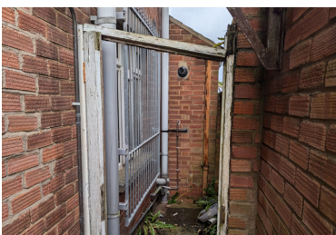
10 - external side passage
