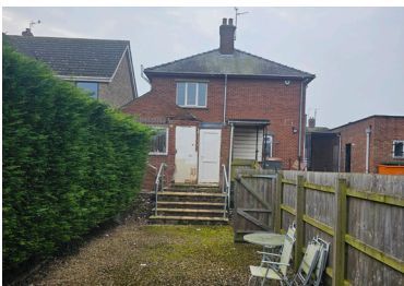
6 - extension stepped access to rear
