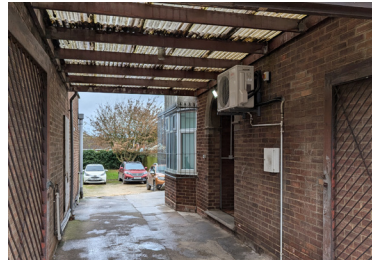
2 - Covered underpass / looking to rear
