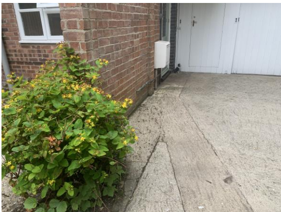
Fig. 11 – Separate building services installed historically.
