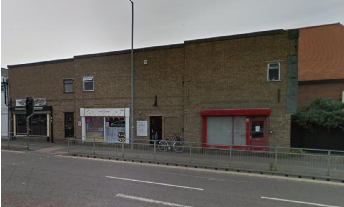
External view from A151 Road
