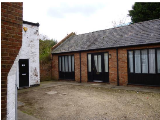
Fig. 05 – Courtyard and single storey rear block.
