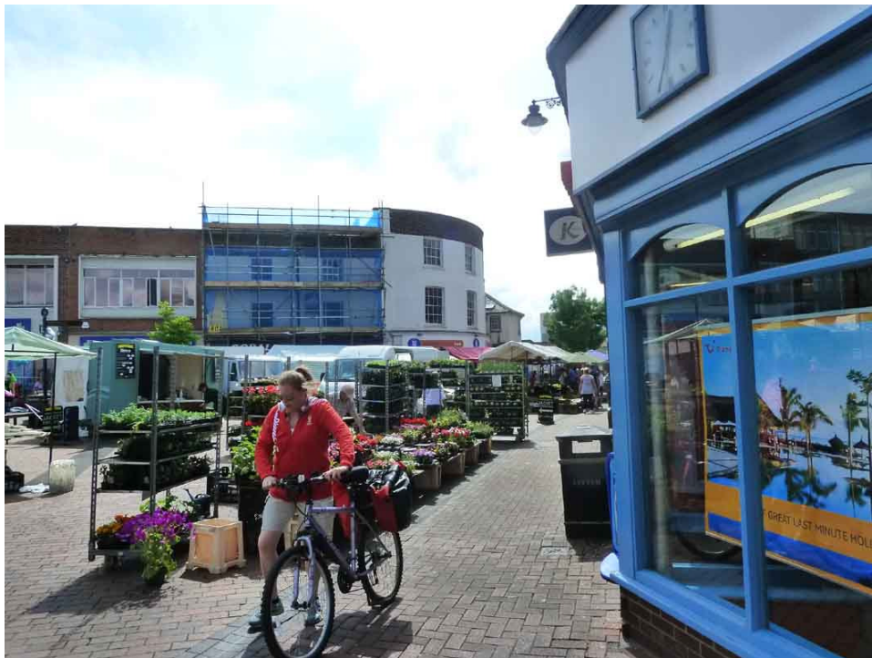
View of subject building from Hall Place, looking south west
