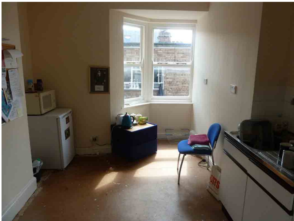
Existing first floor kitchen area to rear of building
