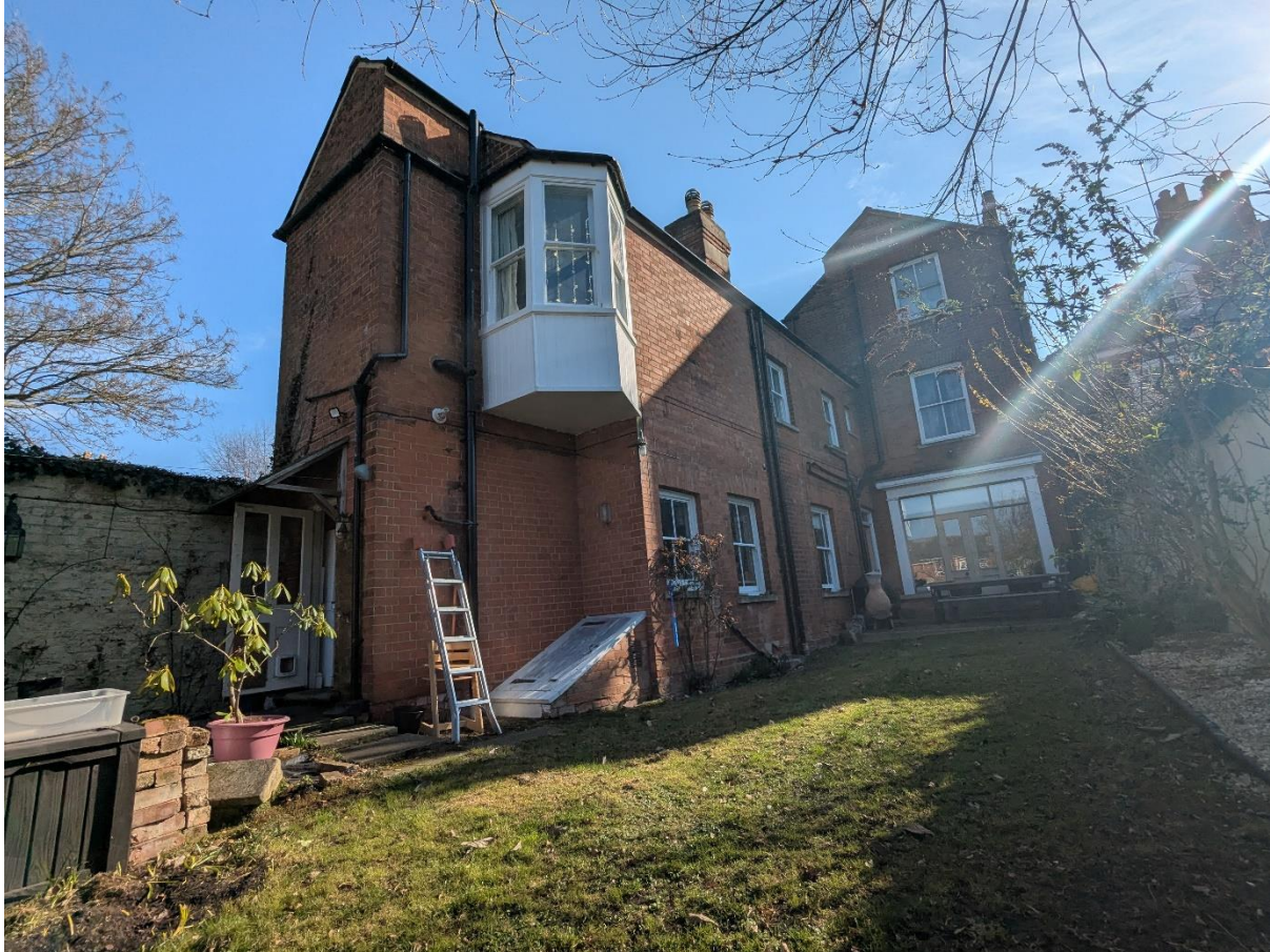
View of rear of existing house
