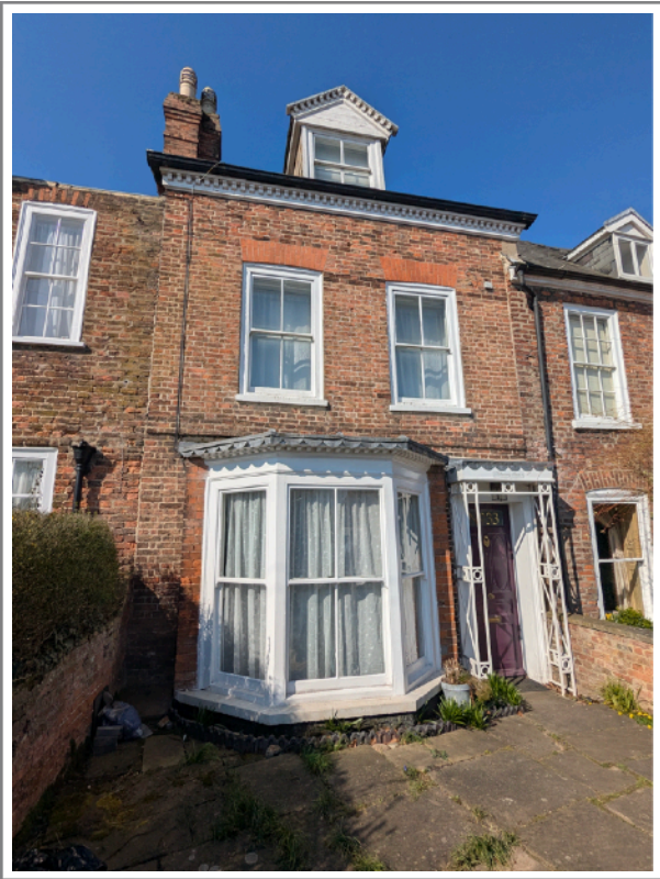
Pic 3: The existing front of the building.
