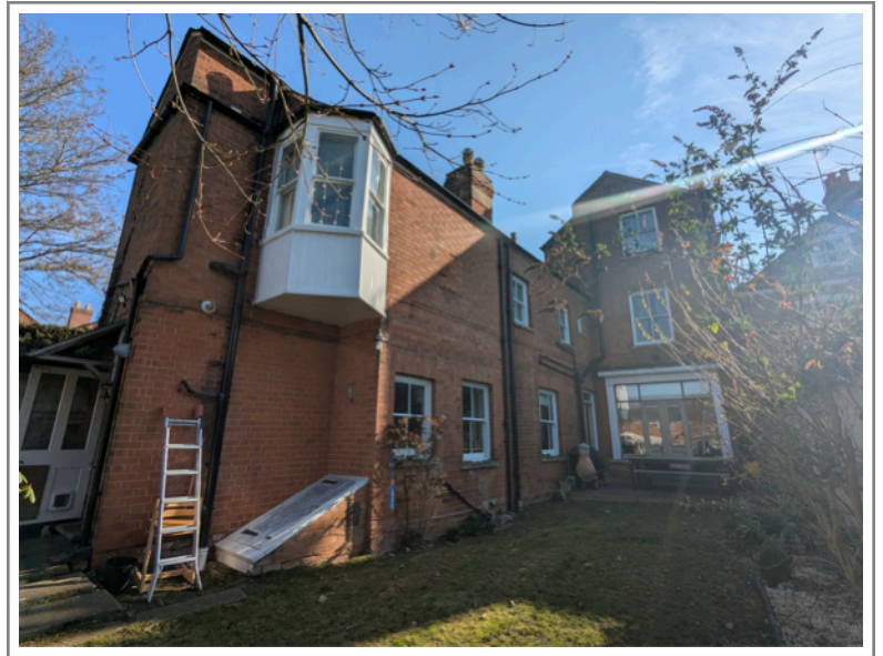
Pic 4: The existing rear of the building.
