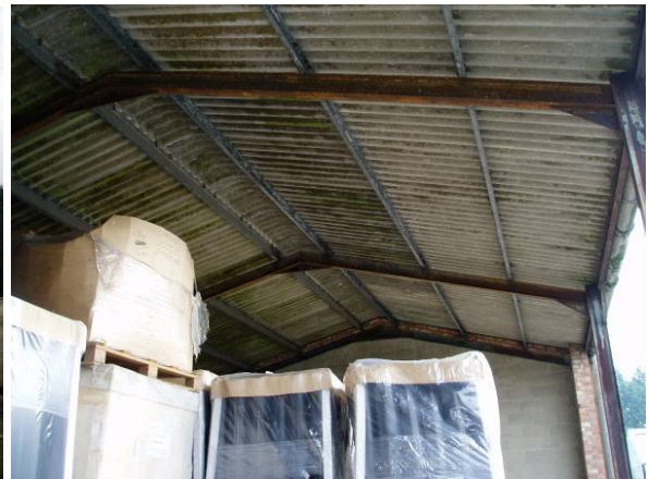
Internal roof of building 10
