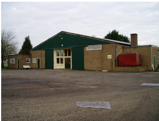
Gallery (south side Building 1)
