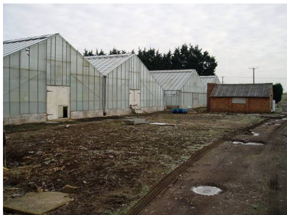
Glasshouses 3 /4 with building 4A
