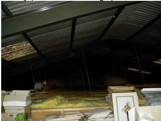
Roof space over Gallery
