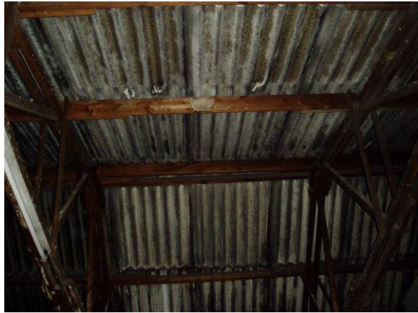
Internal roof of building 9
