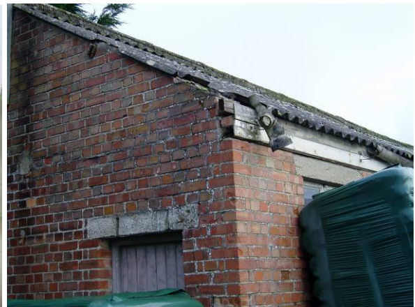
Roof of building 11
