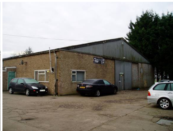
Garage (north side Building 1)
