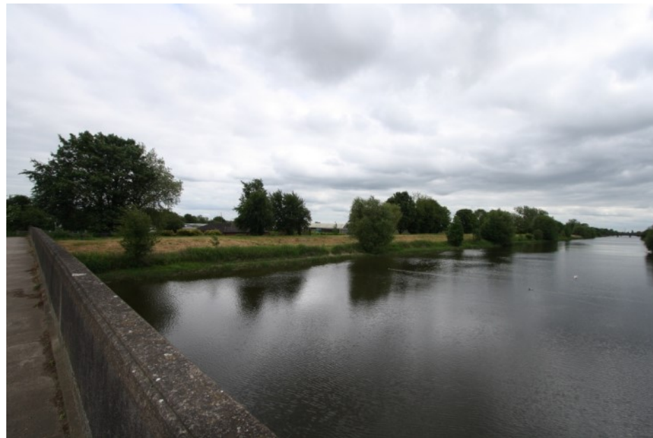
View of Site from Bridge Crossing The Coronation Channel
