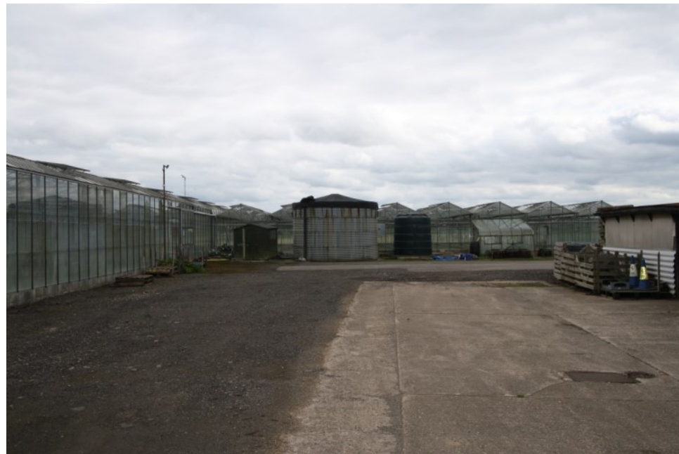
Existing Greenhouses and Surface Water Tank
