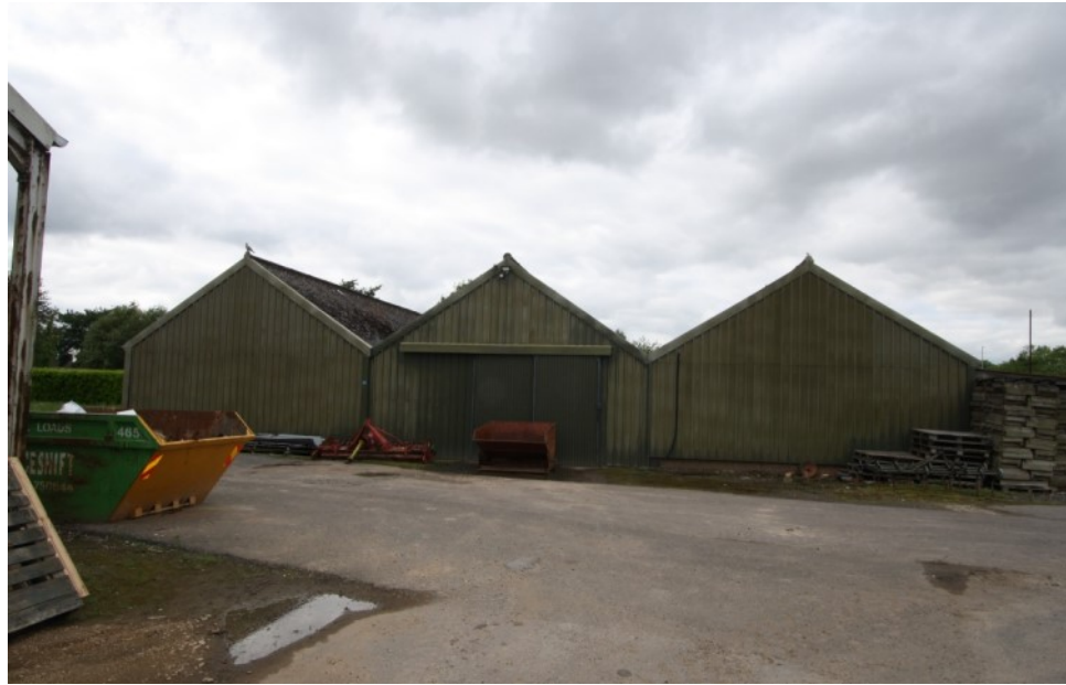
Existing Multi-Bay Barn
