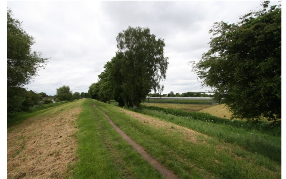
View of Site from Public Footpath Adjacent to the Coronation Channel
