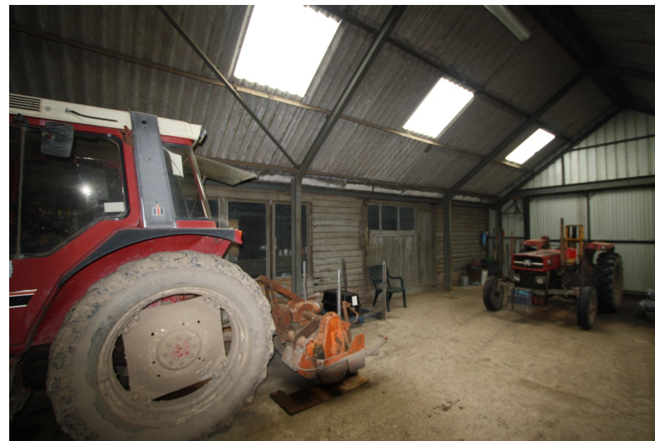
Image Showing Existing Timber Partitions and Cast Concrete Floor
