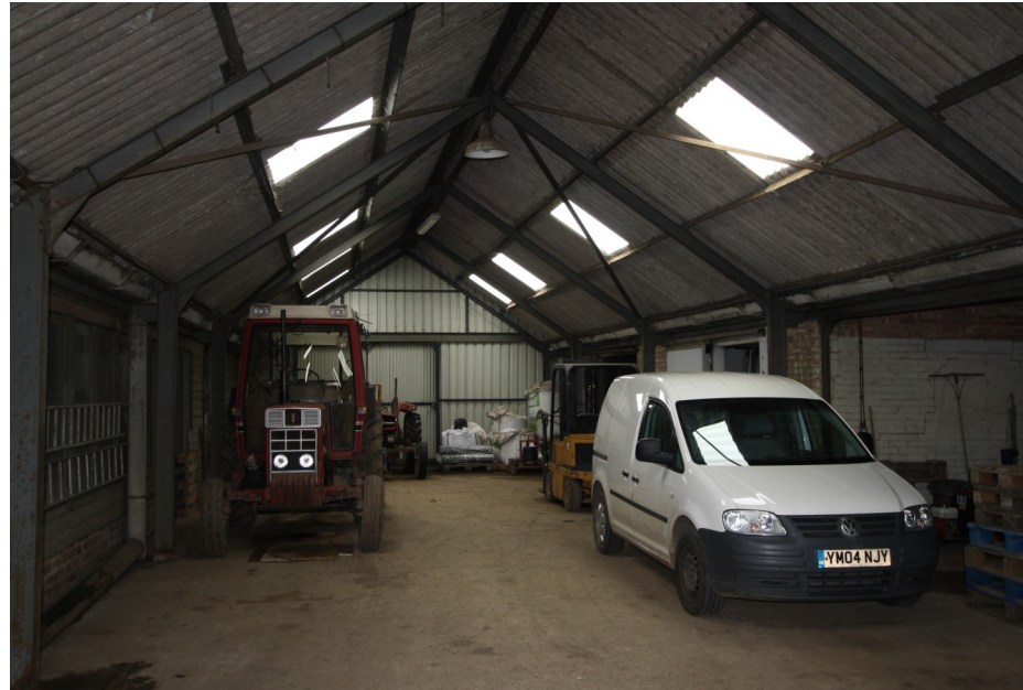
Image illustrating the good condition of the portal frame, roof purlins and sheet material
