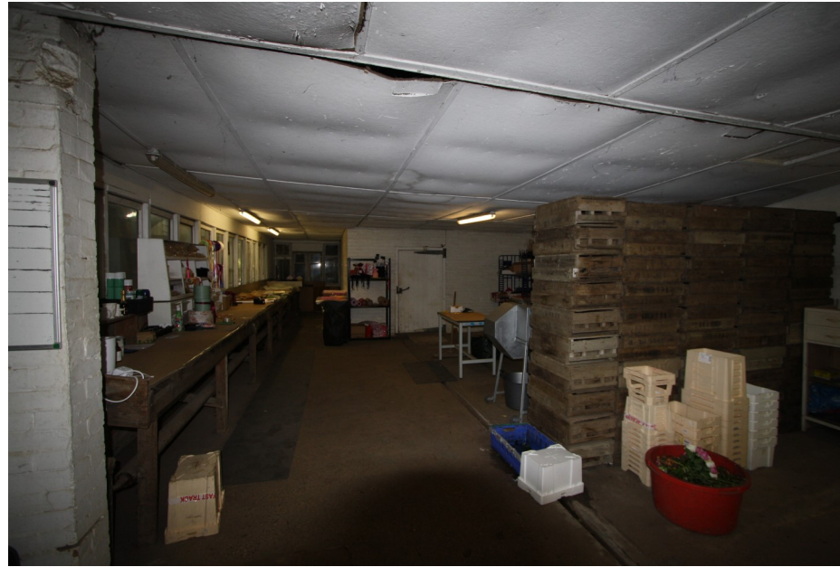
Image Showing Existing Brick Internal Walls and Suspended Ceiling
