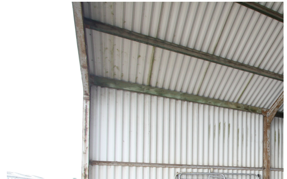
Image Illustrating Steel Profiled Sheet Cladding
