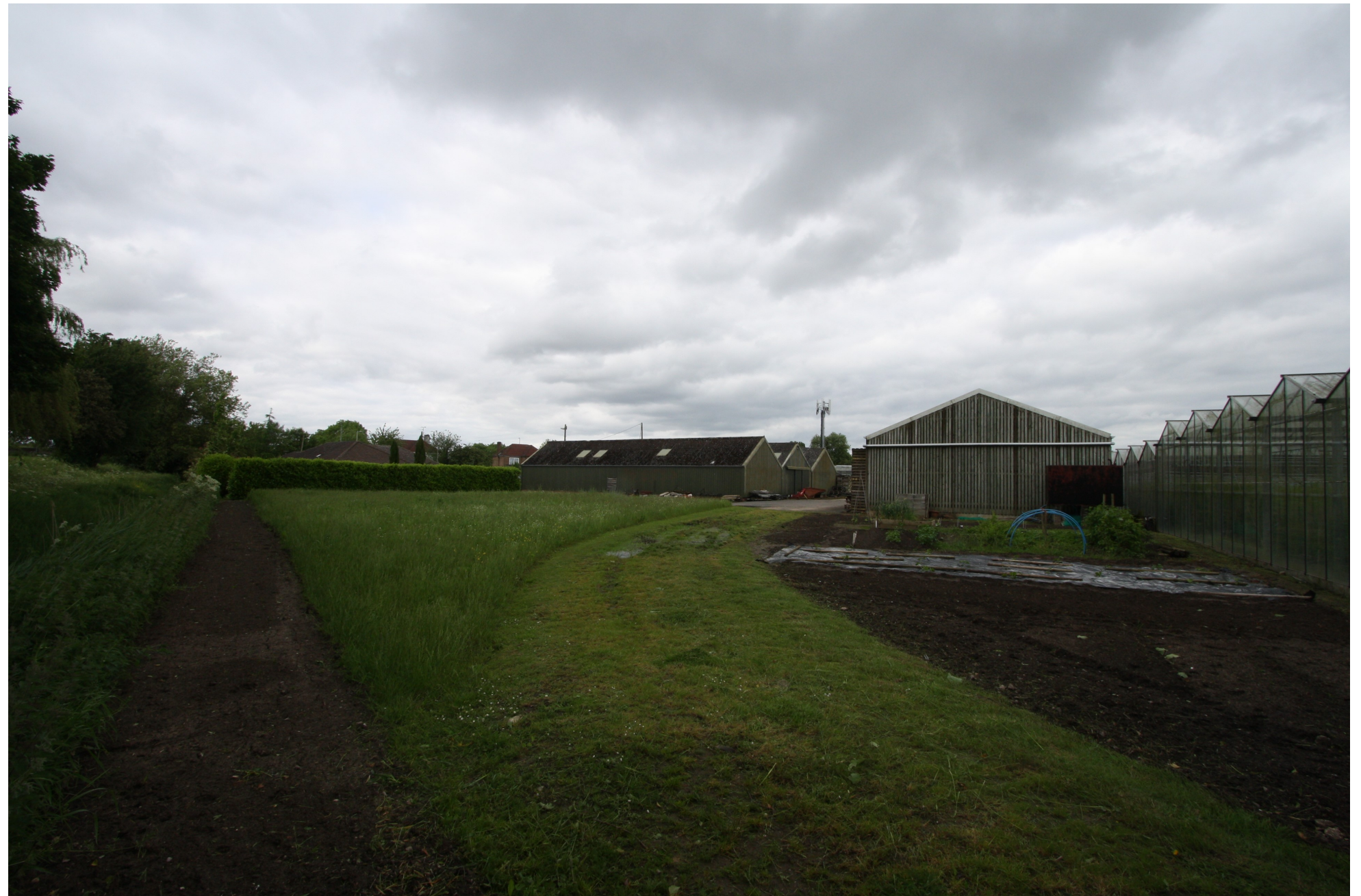
View of West Elevation of Barn B with Barn in the Bakground
