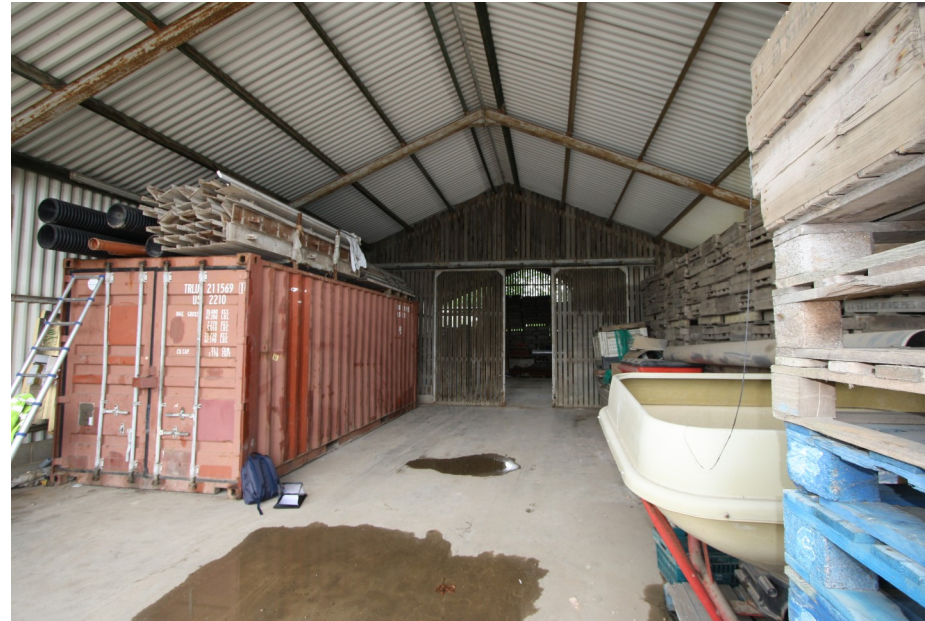
Image Showing Timber Internal Partition, Doors and Cast Concrete Floor
