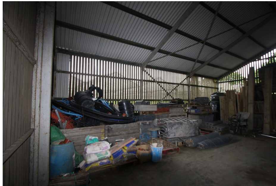
Image illustrating the Excellent condition of the portal frame, roof purlins and sheet material
