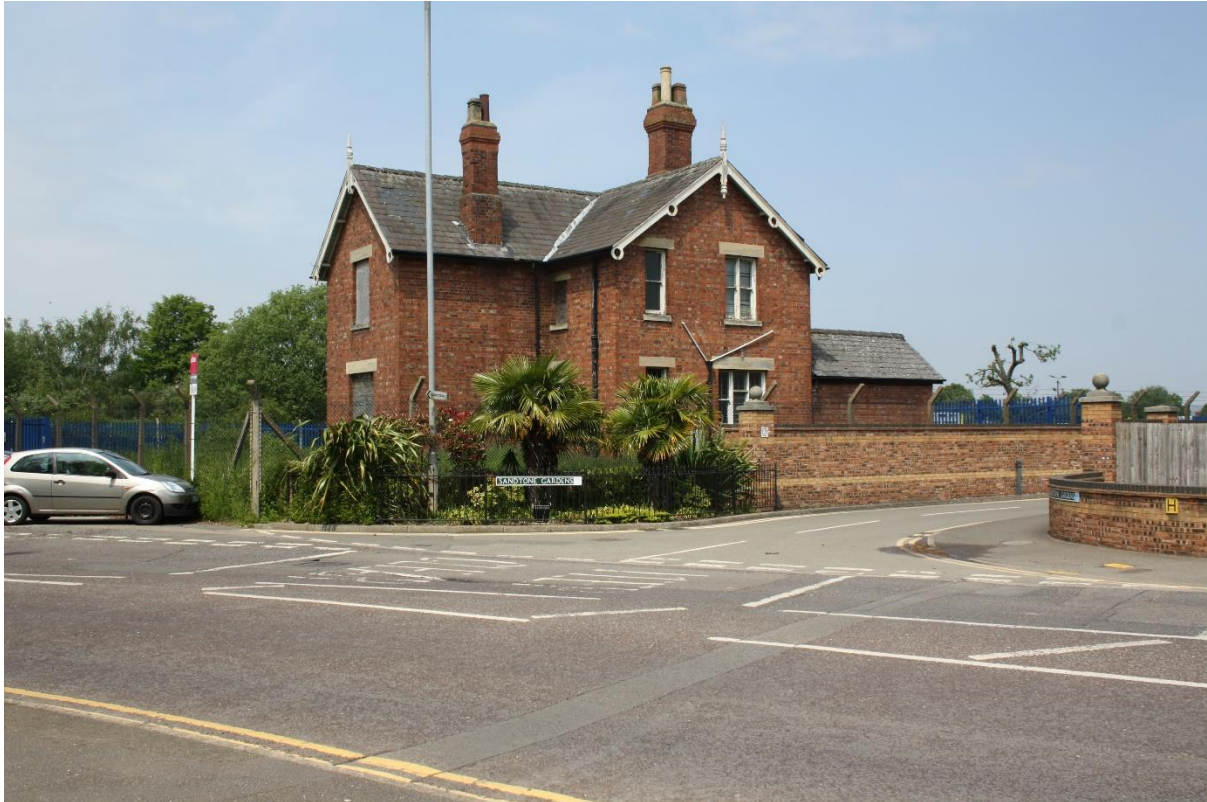
View of development site from Kings Road
