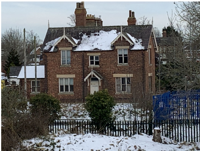
View of Station House from the West – The entire building is to be demolished.
