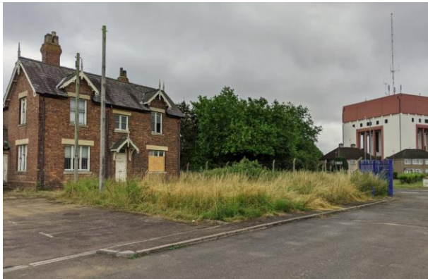
Station House and Chatterton Tower
