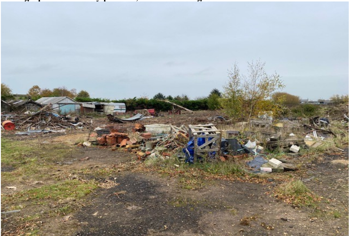
Photograph 2 – Westerly position; stored building materials
