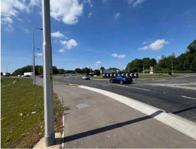
View of Springfields Roundabout
