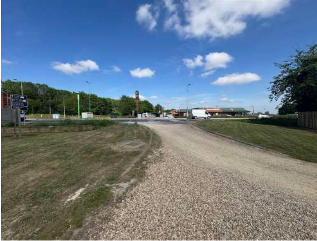
Looking north from existing site entrance
