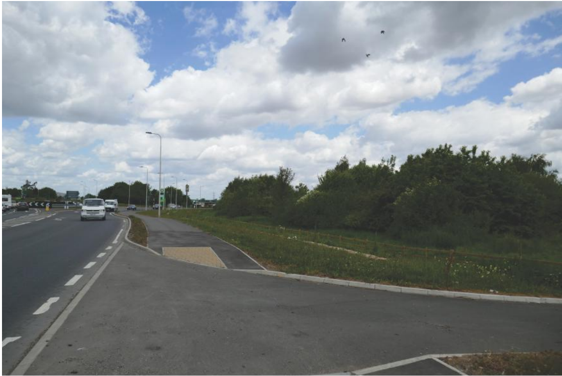
Pl. 7 View north from south-west corner of application site
