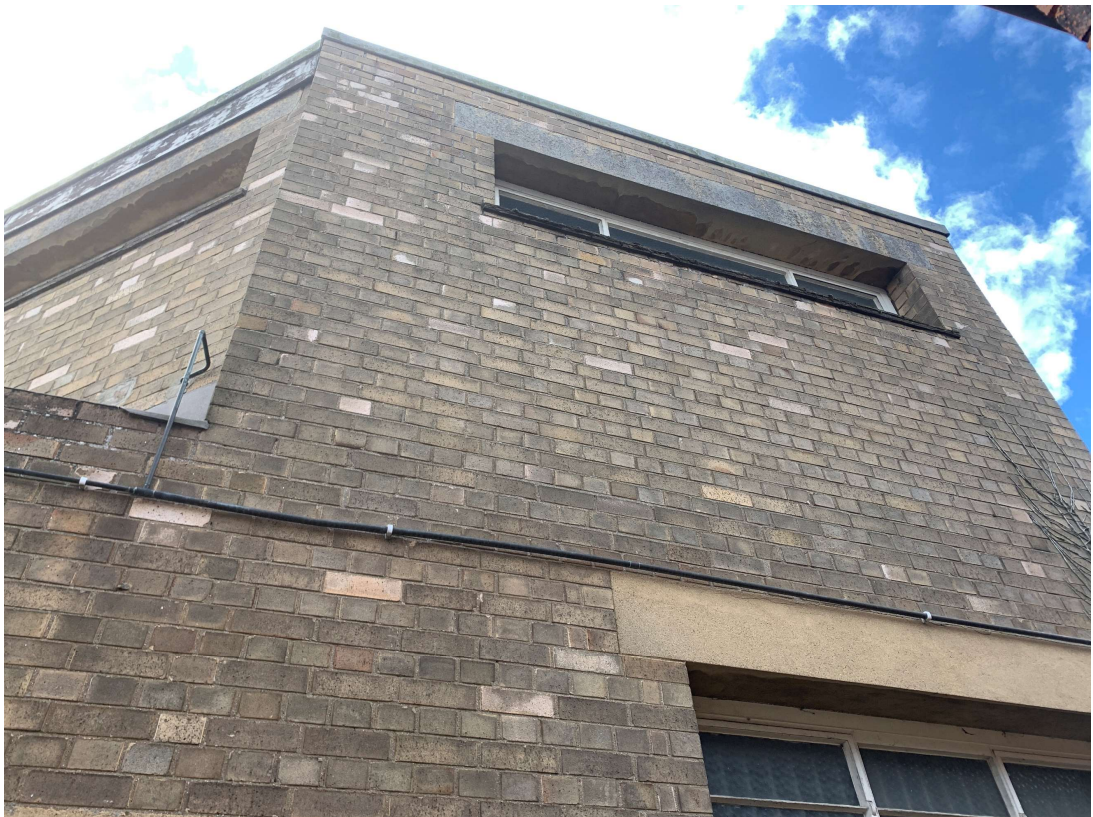
Figure 3: Present day rear extension
