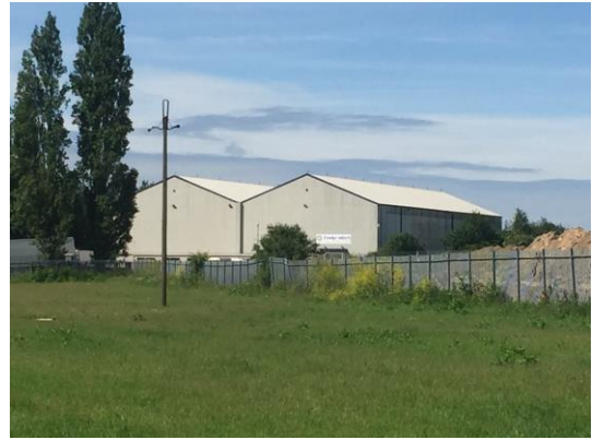
Fig. 04 – 24 West blocks (warehouse 2).
