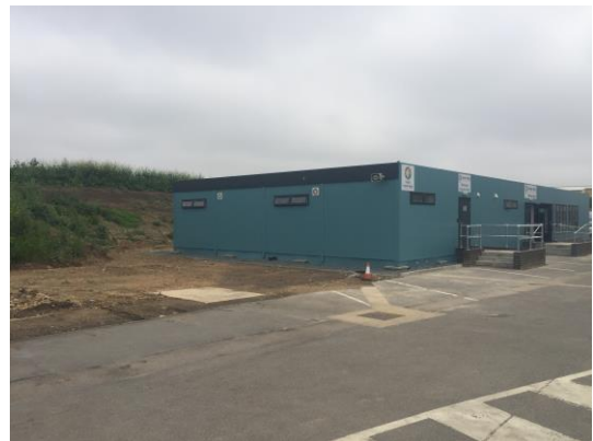
Fig. 06 – Recently erected staff welfare block
