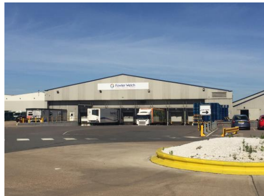
Fig. 02 – Main central warehouse block.
