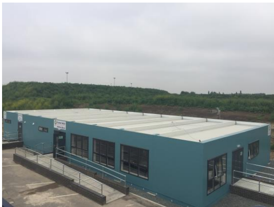
Fig. 05 – Recently erected staff welfare block.
