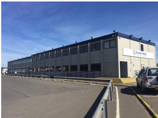
Fig. 01 – Office administration block.
