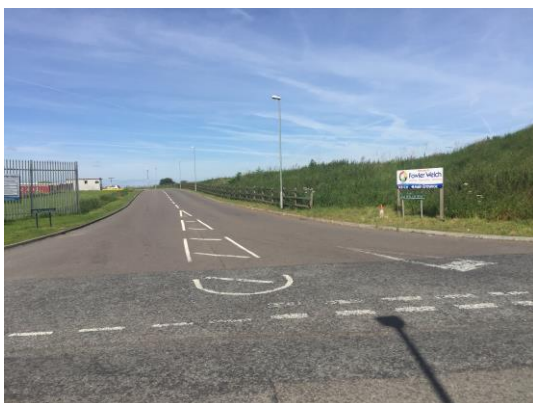
Fig. 12 – Main lorry access on West Marsh Road.
