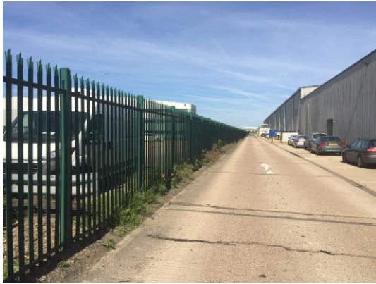
Fig. 16 – Boundary on south-west side of site.
