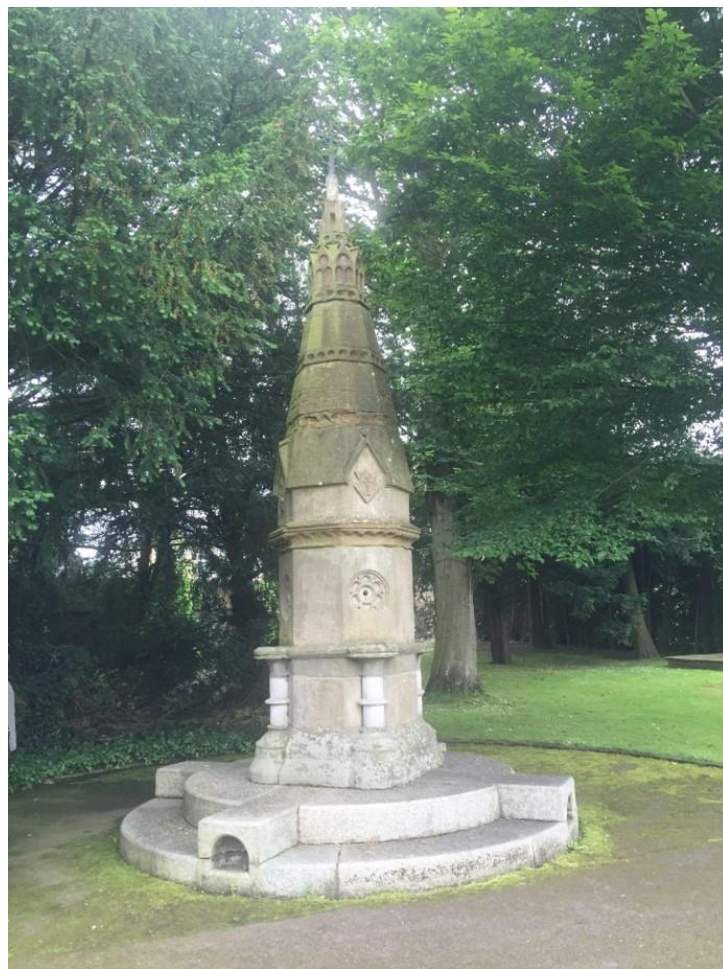
Plate 1: The fountain prior to dismantling
