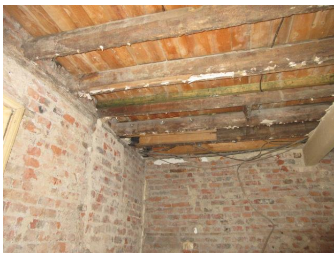
Photograph # 14 (Room 1 / Room 2- Typical Floors over)
