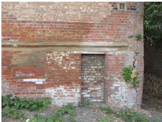
Photograph # 3 (See Area 1 – Drawing 6618-100) (Rear Projection – Rear Gable Elevation)
