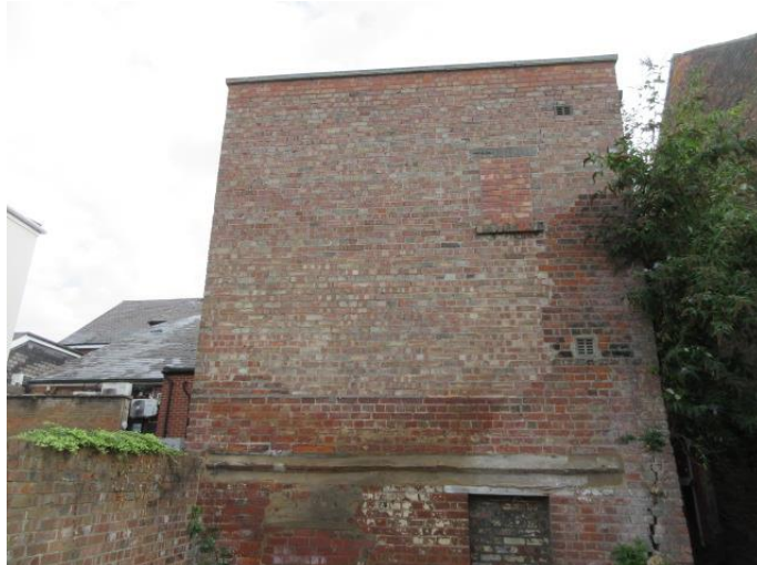
Photograph # 2 (See Area 1 – Drawing 6618-100) (Rear Projection – Rear Gable Elevation)
