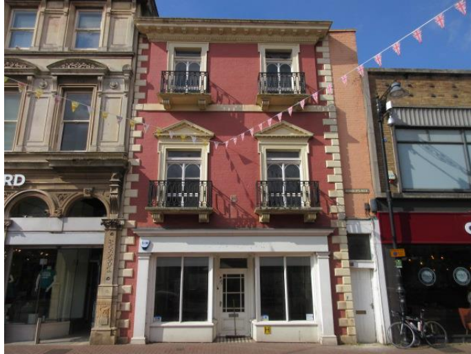
Photograph # 1 (Front Elevation)
