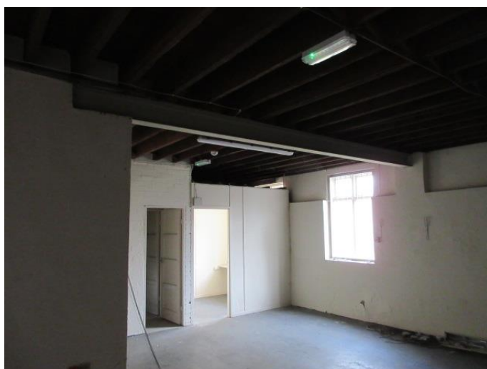
Photograph # 18 (Rear Projection Ground Floor)
