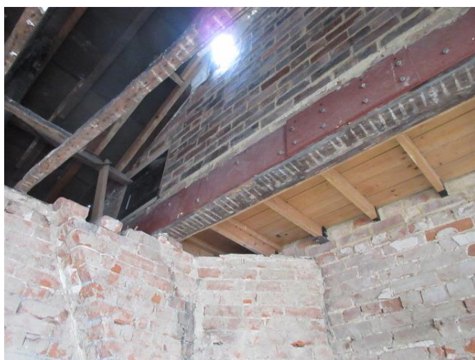
Photograph # 15 (Room 4 – Existing Chimney Support)
