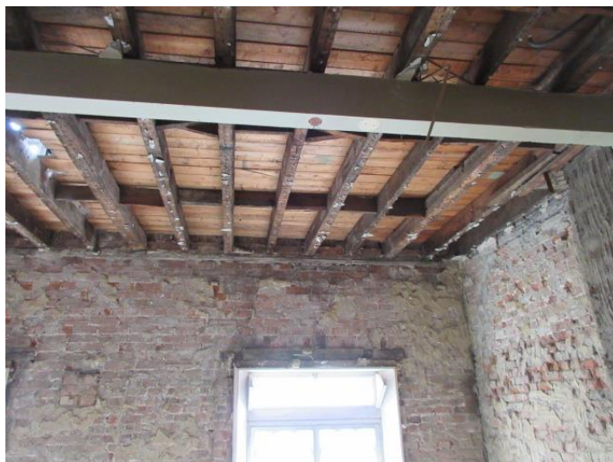
Photograph # 13 (Room 1 / Room 2- Typical Floors over)
