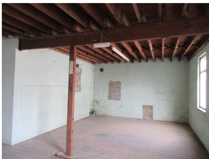
Photograph # 19 (Rear Projection First Floor – Room 7)
