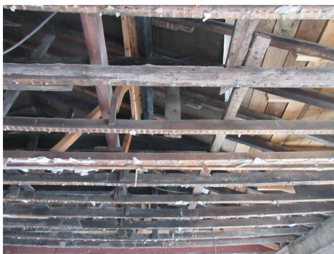
Photograph # 17 (Room 4 – Existing Roof)
