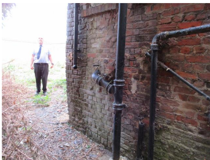
Photograph # 5 (See Area 1 – Drawing 6618-100) (Rear Projection – Flank Elevation / Corner of Rear Gable)
