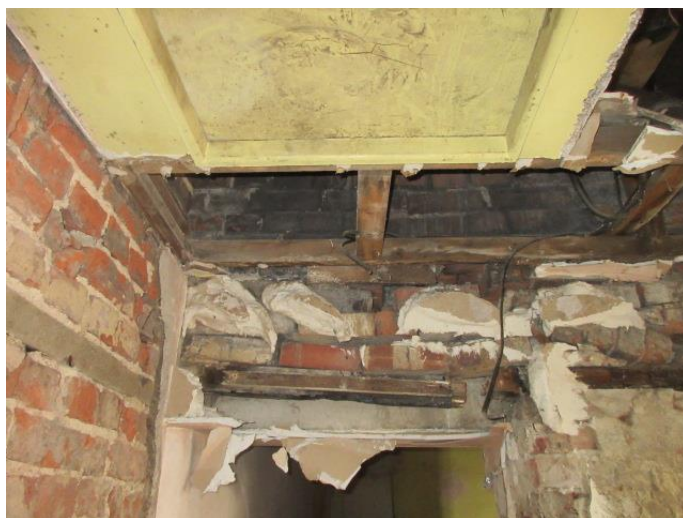
Photograph # 11 (See Area 7 – Drawing 6618-100) (Room 6 / Landing)
