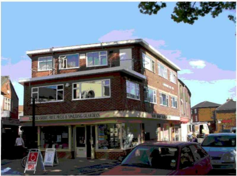
4 The Crescent (Lincolnshire Free Press) Three storey building, height to eaves 8.2m Plot width / frontage 14m (corner plot) External walls in brown / red facing brick Shop fronts and windows in timber 300mm eaves overhang in timber Flat roof with extended eaves
