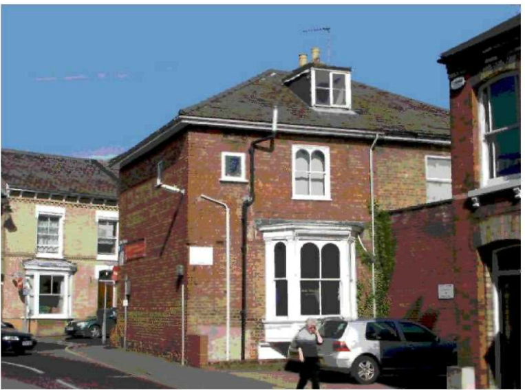
30 & 31 The Crescent (rear) Three storey building (inc. basement) in brick with pitched roof
