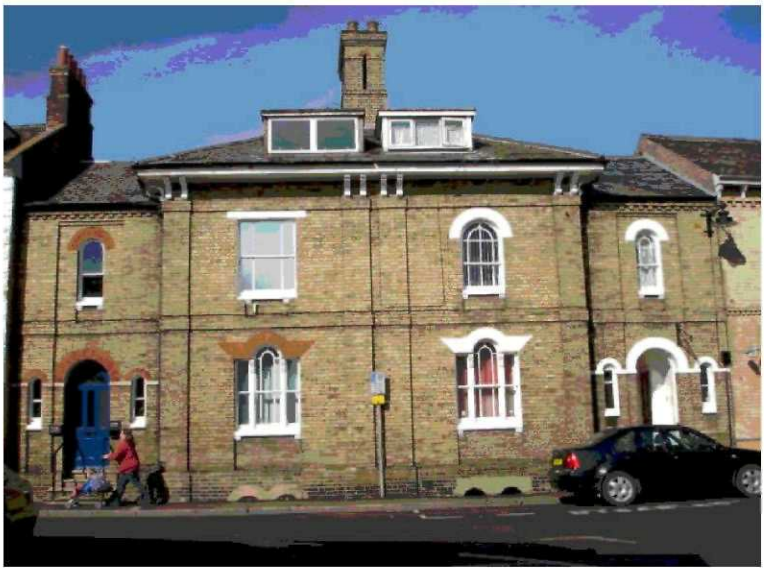
9 & 10 The Crescent Four storey building (inc. basement), height to eaves 7.0m Plot width / frontage approximately 8.0m (divided by projecting bay) External walls in buff brick with red gauged brick around openings Doors and windows in timber, vertical sliding sash style 400mm eaves overhang in timber Pitched roof with slate finish
