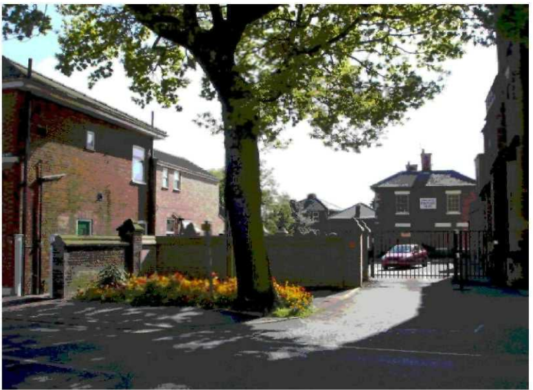
Former Police Station
